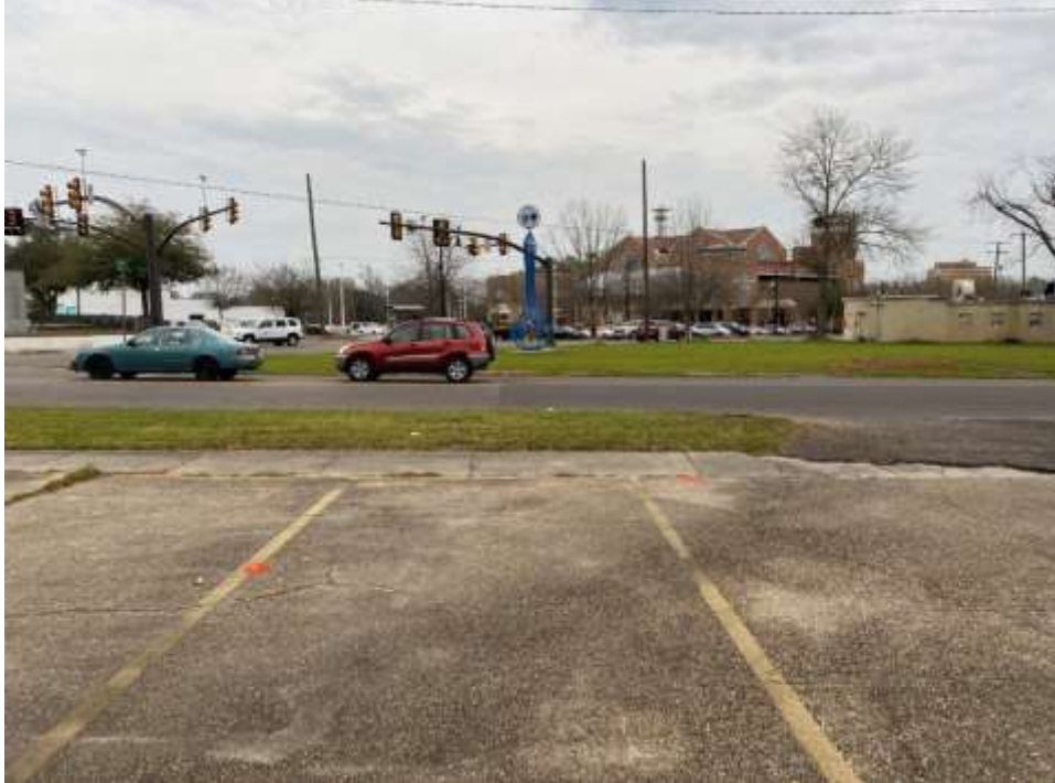
View of paving in R.O.W
