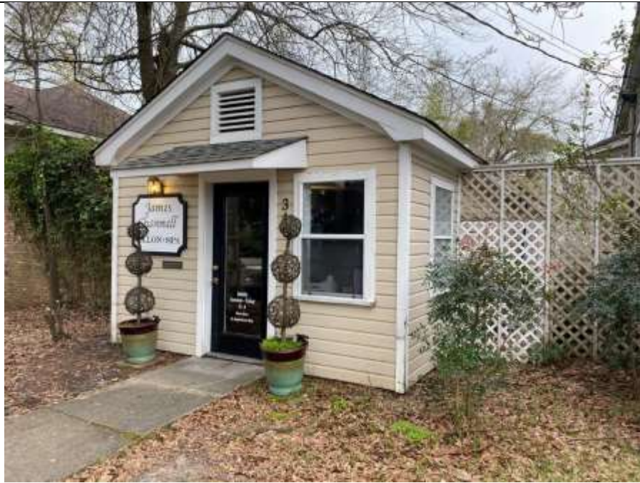
Detached rental unit along East side of building.
