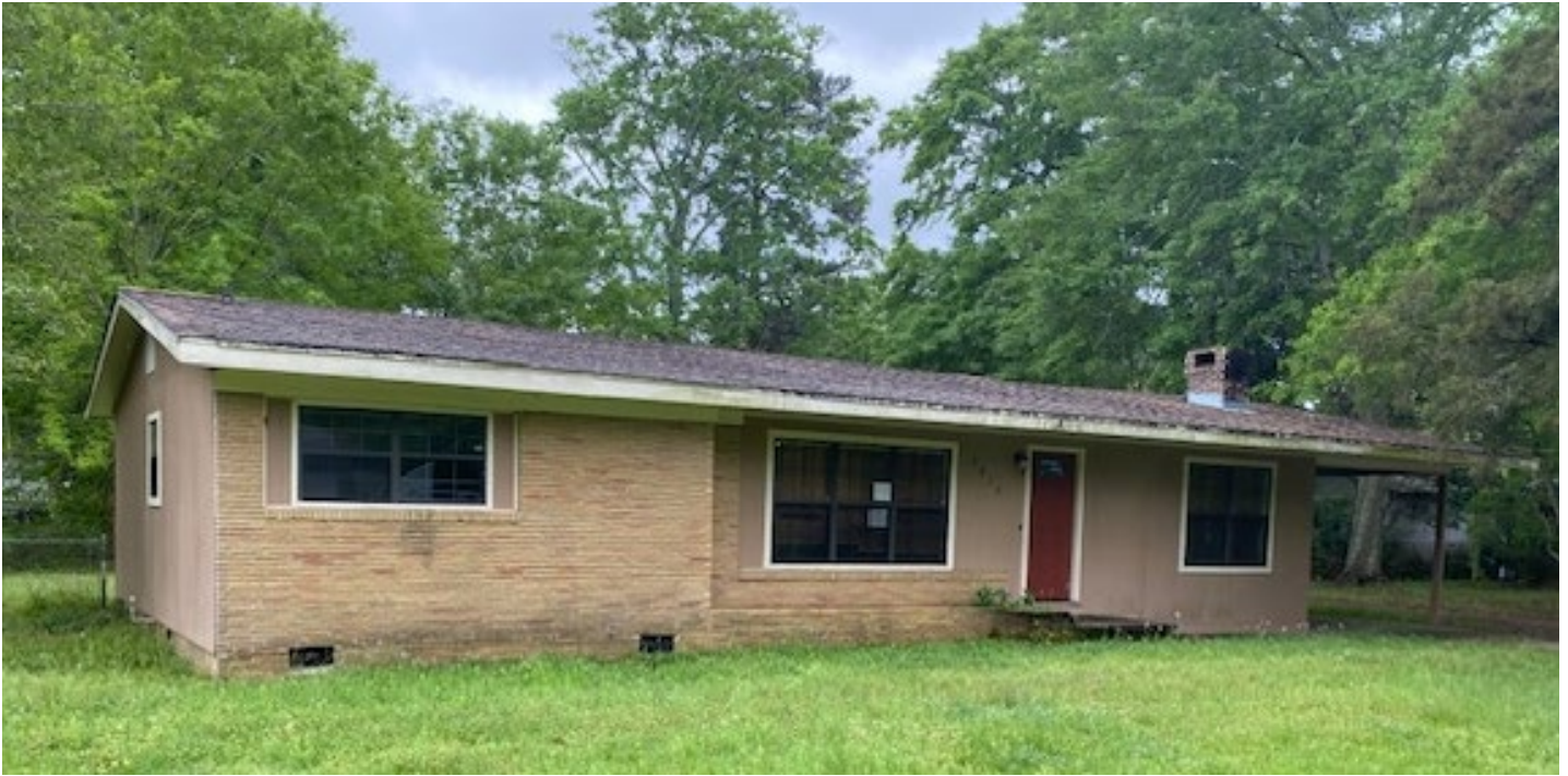
Existing House – April 2026
