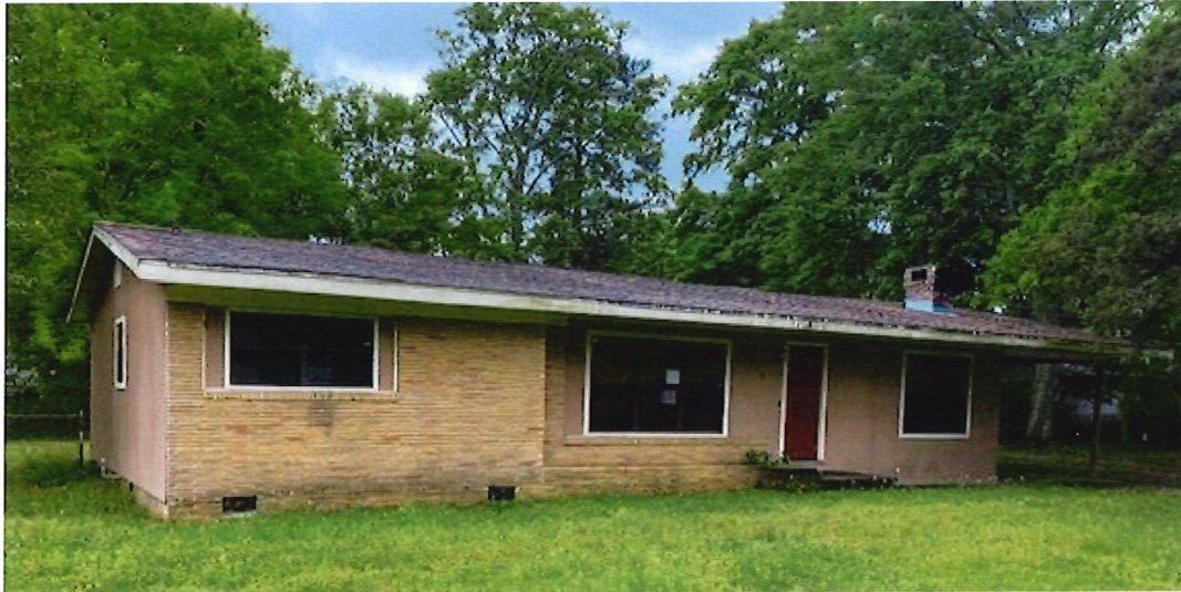
Existing House – April 2026
