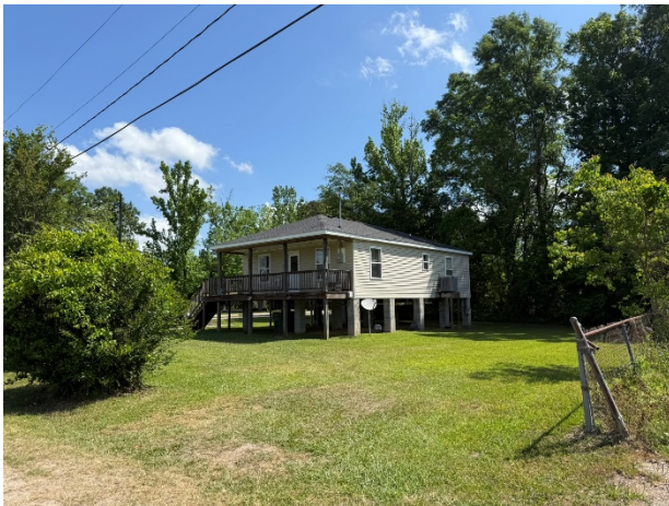
Surrounding Area Image- Example of a nearby structure elevated above the BFE
