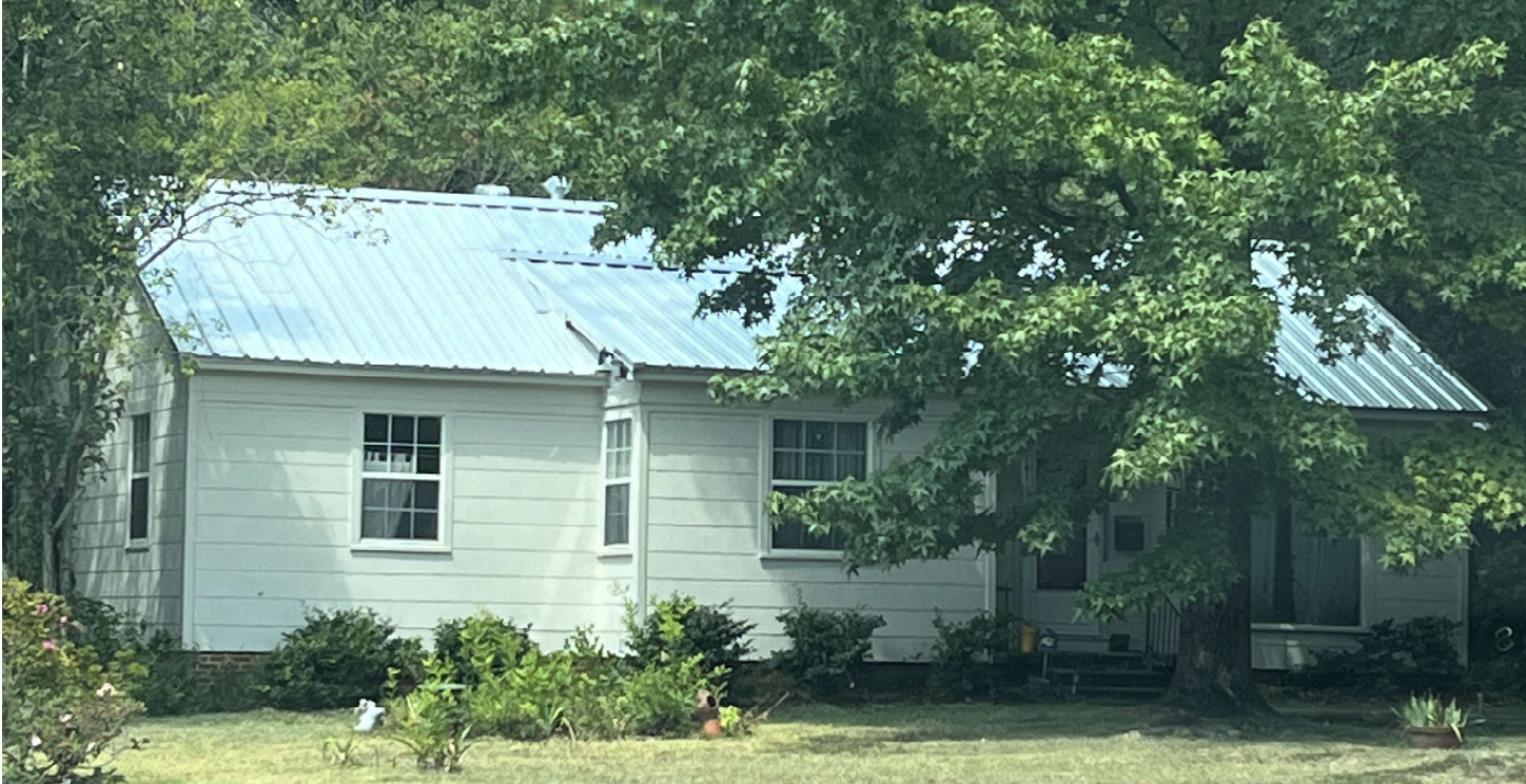
Current view of roof with metal panels installed
