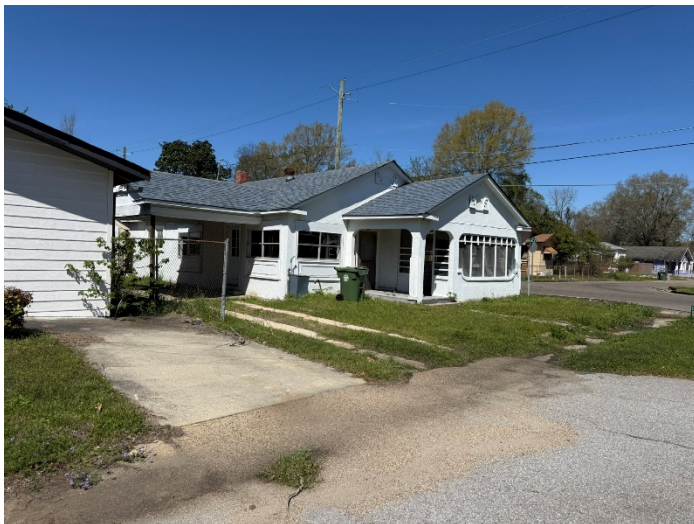
Property / Surrounding Area Image
