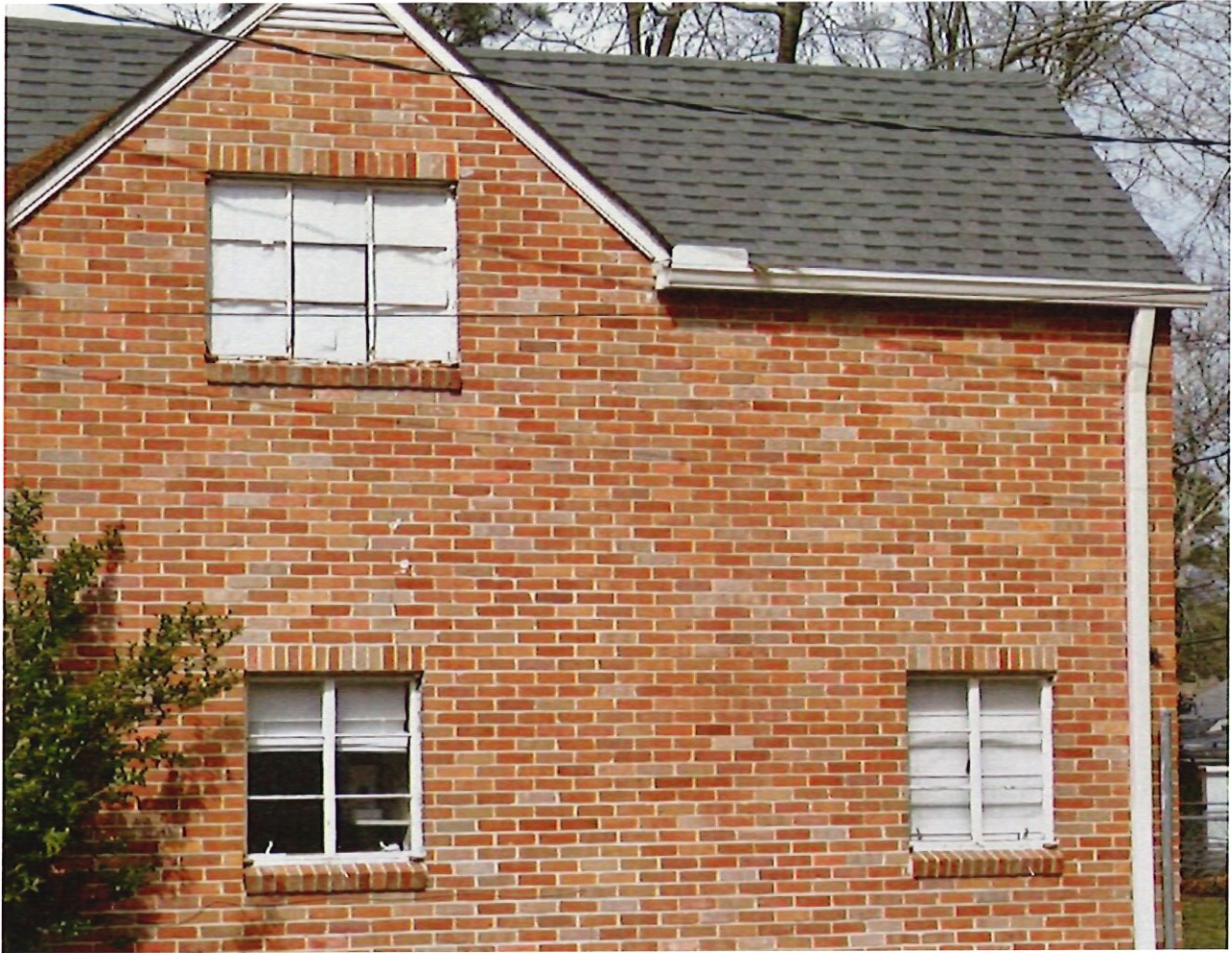
Street view showing existing windows on S facade
