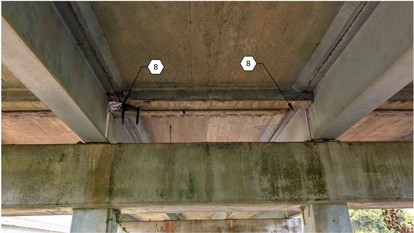
UNDERSIDE OF BRIDGE SHOWING CAP, BEAMS, SLAB, AND DROP SLAB
