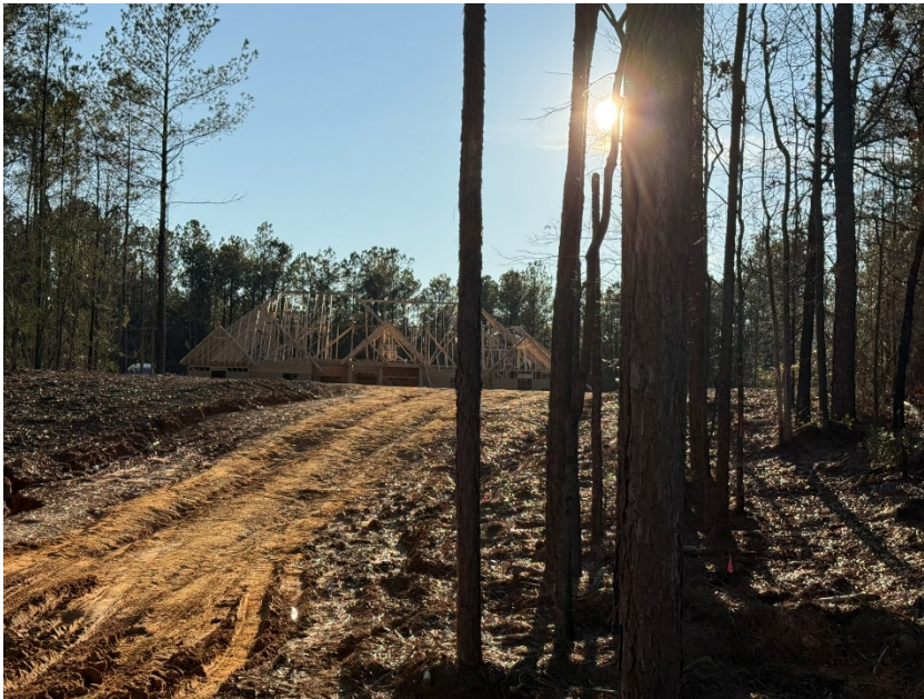
Property Area Image- Home Under Construction
