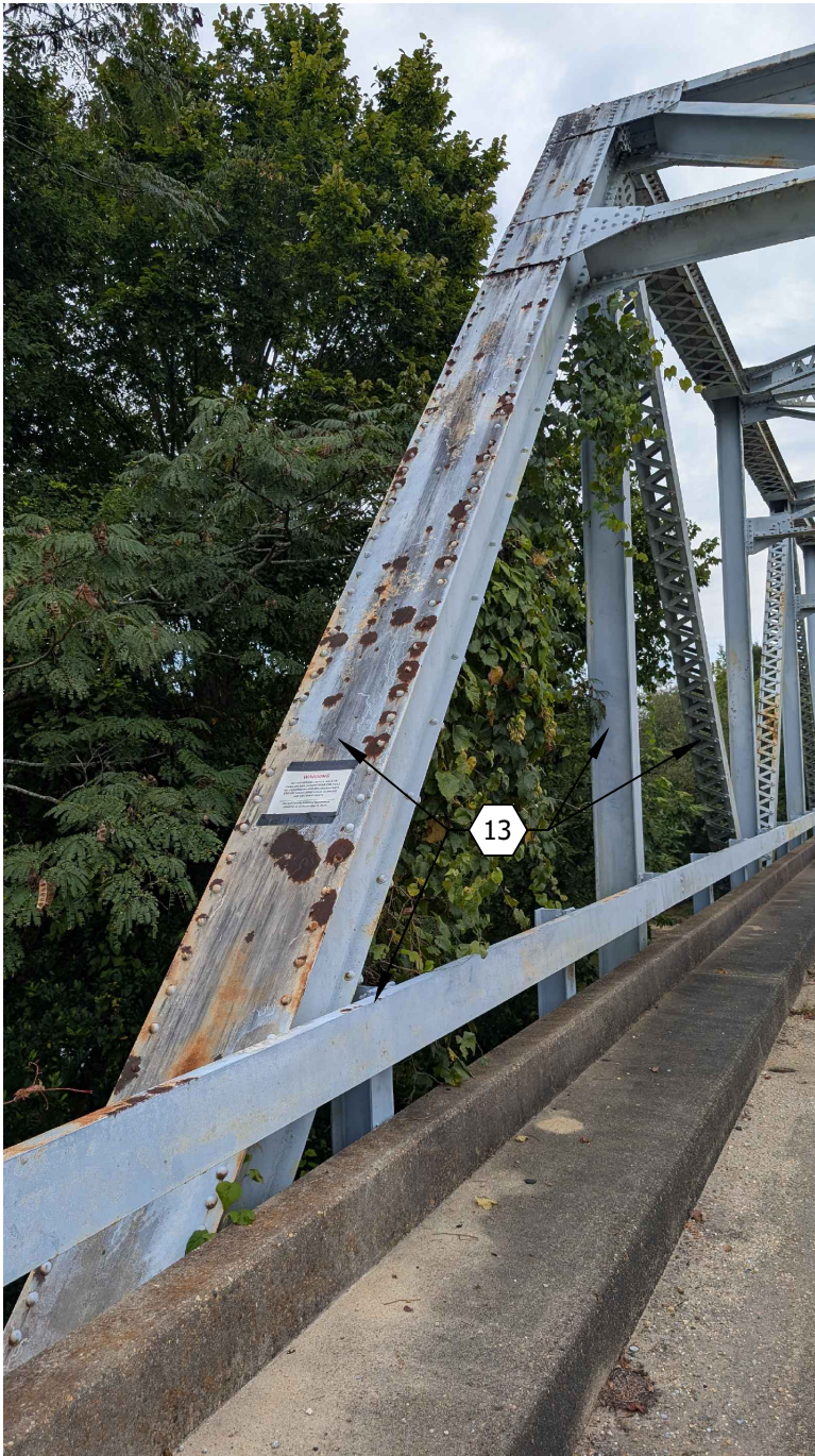
END POST AT SOUTHWEST CORNER OF TRUSS
