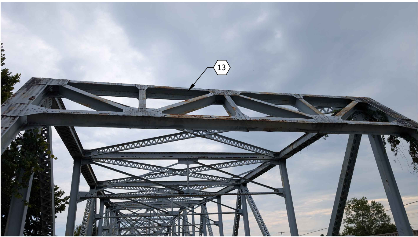
PORTAL FRAME AT SOUTH END OF TRUSS
