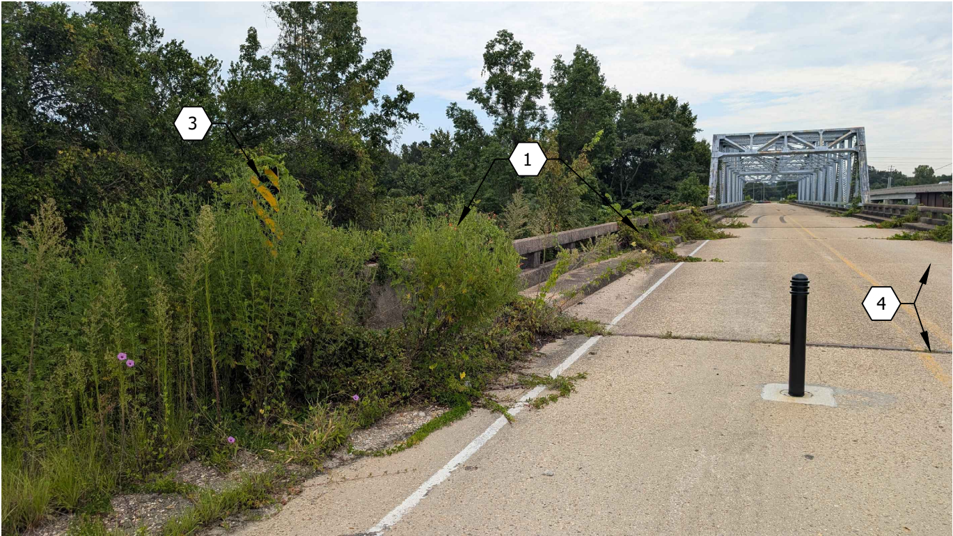
SOUTHWEST CORNER OF BRIDGE
