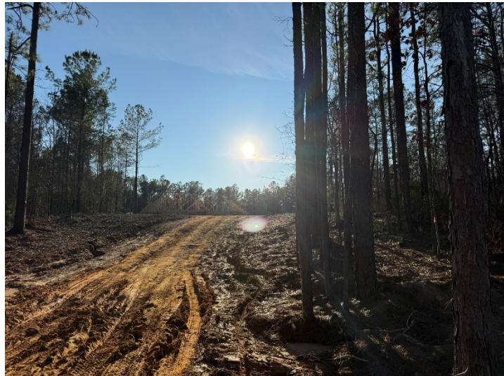
Property Area Image- Home Under Construction
