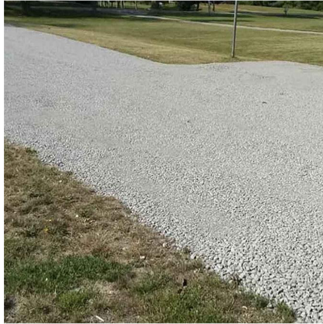
Potential Example of "Crusher Run" Driveway
