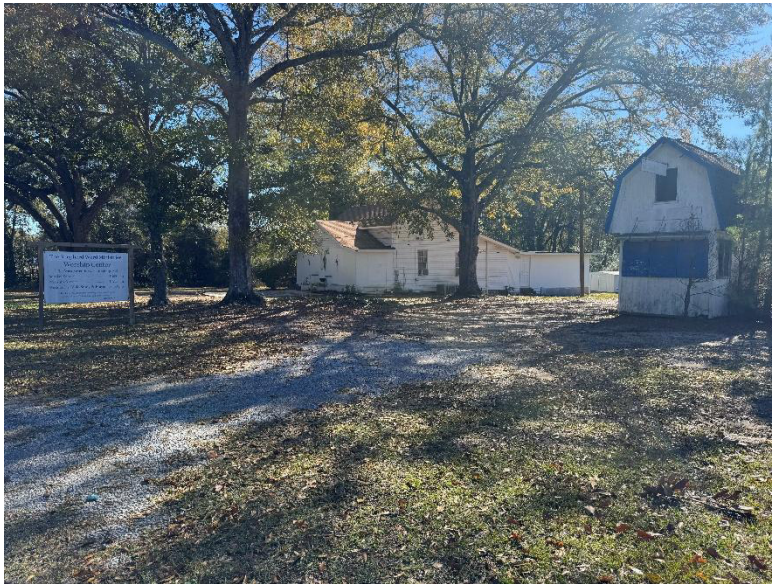
Surrounding Area Image- Adjacent property (east of Subject Property)
