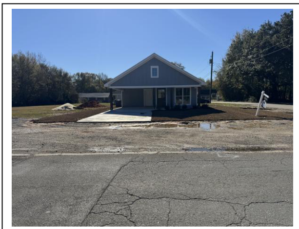
Property / Surrounding Area Image- Adjacent Newly approved subdivision and homes
