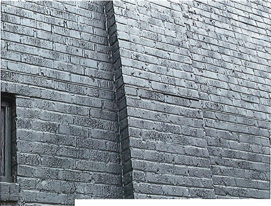
South Wall—masonry cracking and wall deflection near parapet
