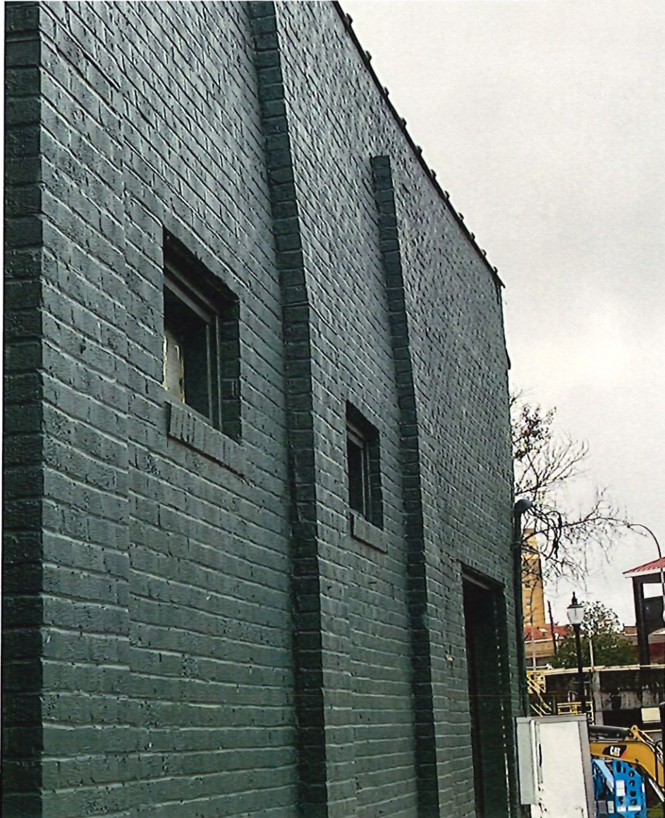
South Wall—masonry cracking and wall deflection near parapet
