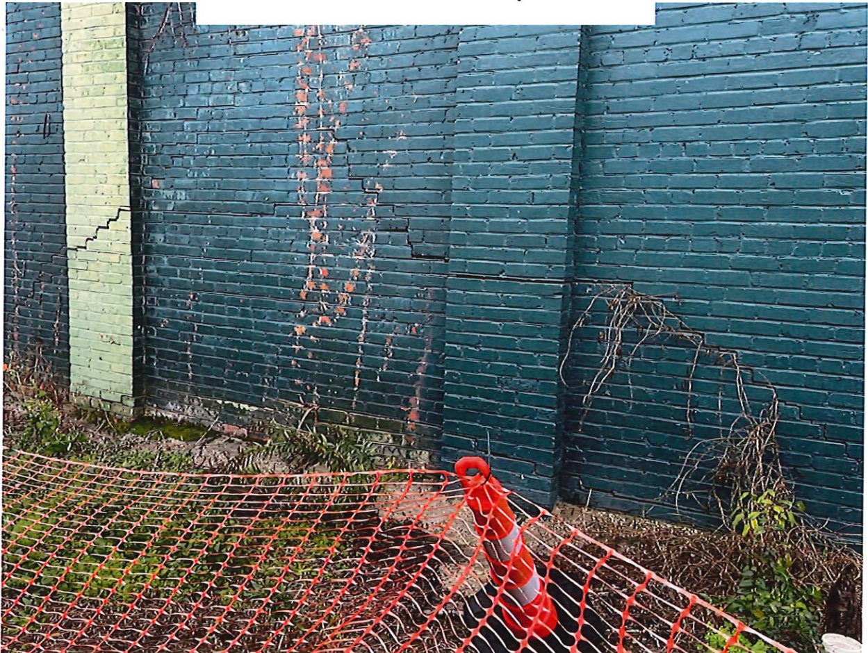
North Wall—structural separation
