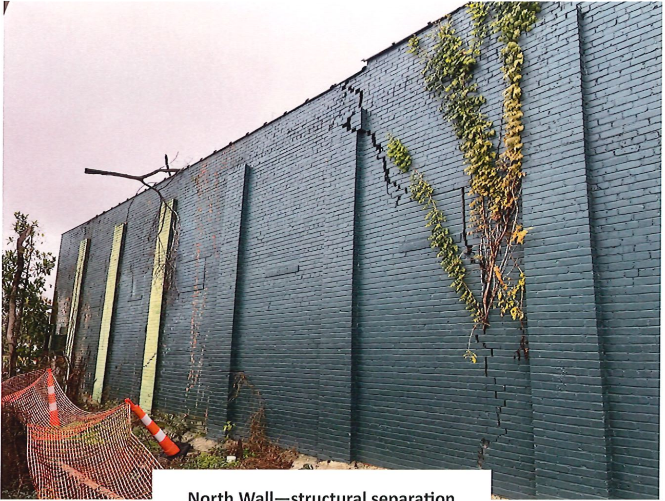
North Wall—structural separation
