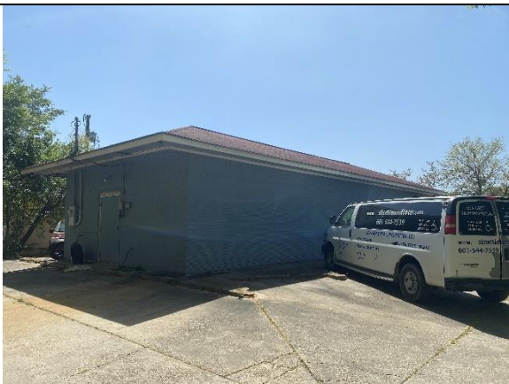
Rear of the building
