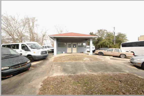
Overall Front View
