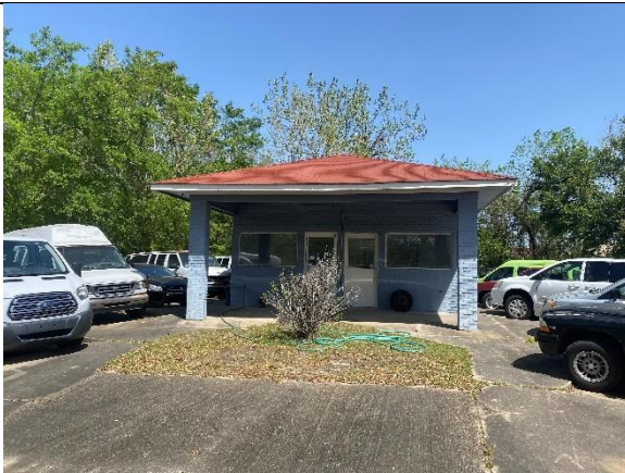
Front of building
