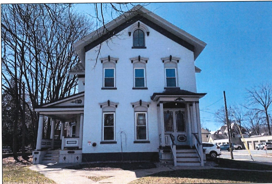
Photograph 7. Overview of Resource 11304.000138, camera facing west. A. Nestor 04/01/2025.
