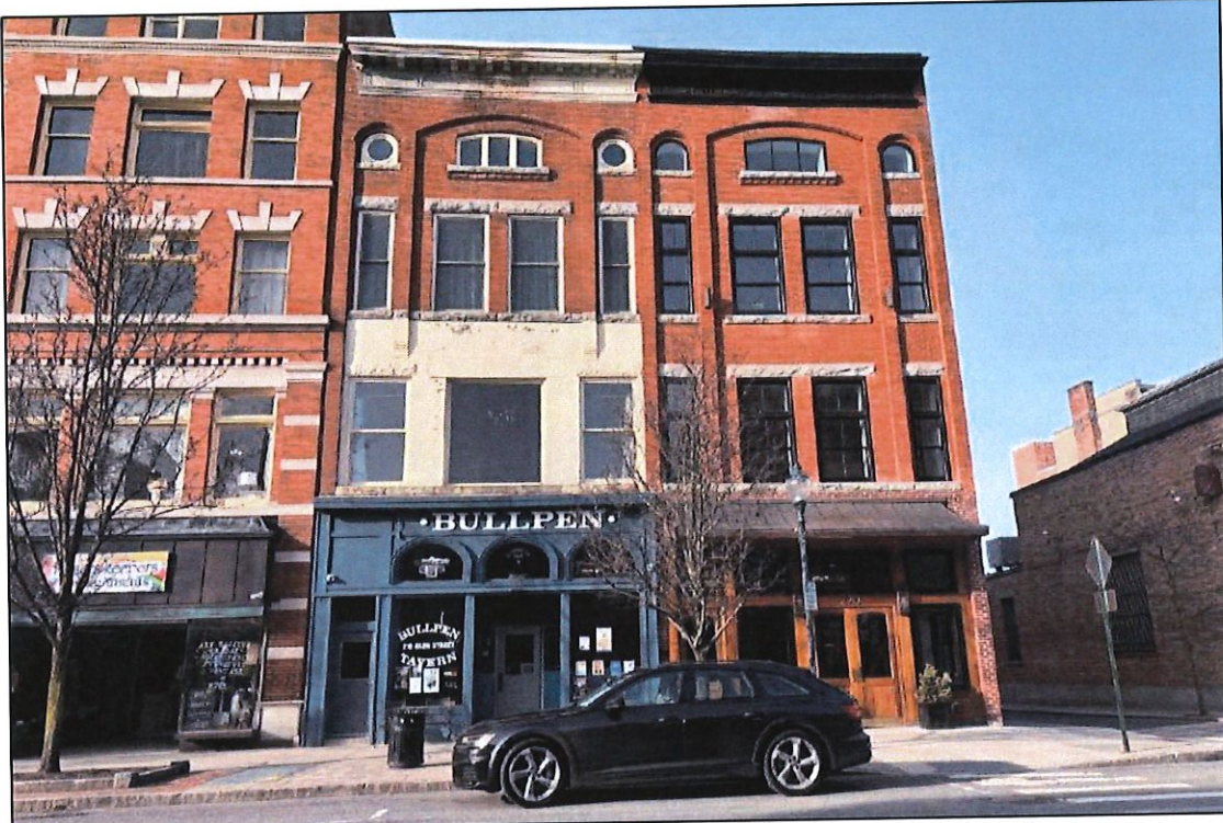
Photograph 23. Overview of Resource 11304.000188, camera facing west. A. Nestor 04/02/2025.
