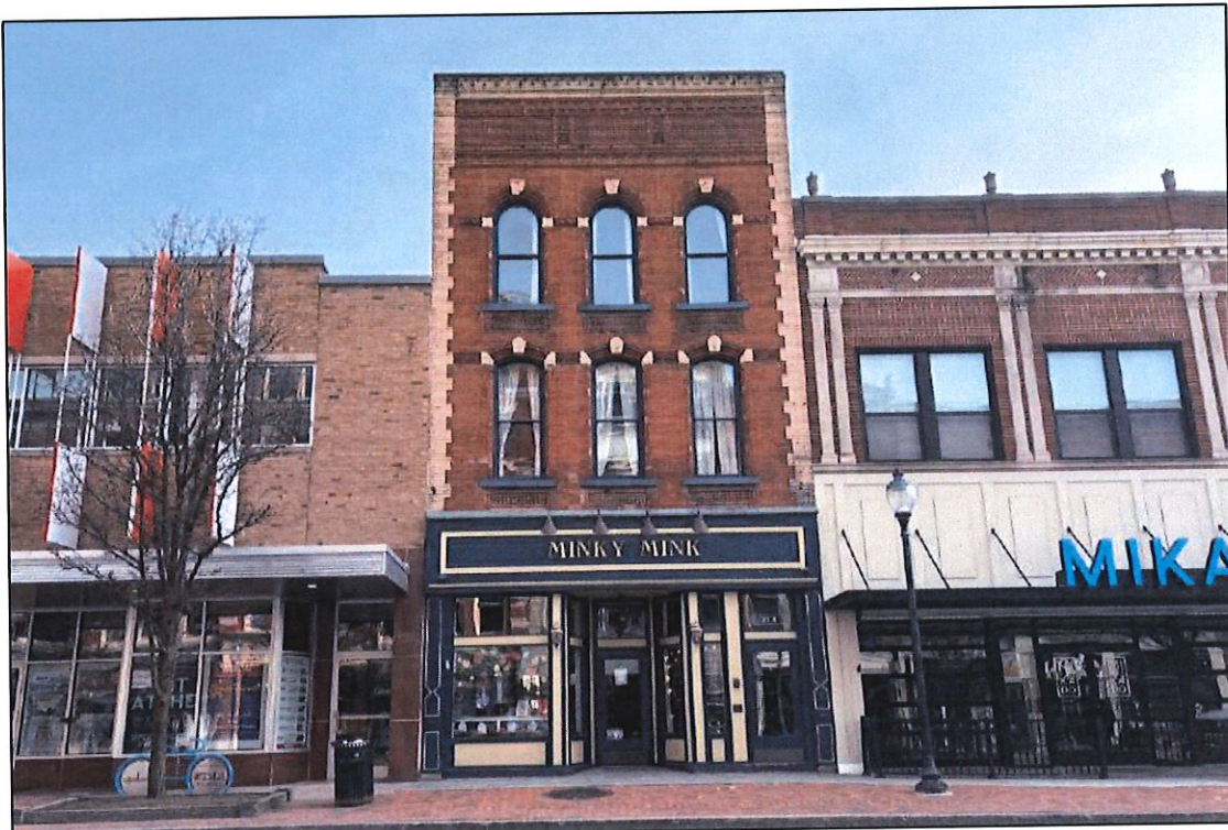
Photograph 19. Overview of Resource 11304.000185, camera facing west. A. Nestor 04/02/2025.
