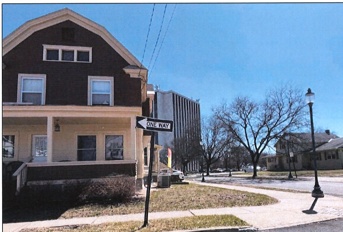
Photograph 112. View toward collocation from Resource 11304.000372, camera facing south. A. Nestor 04/01/2025.
