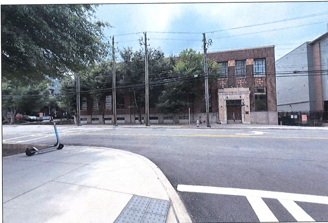
Photograph 17. Overview of Resource 249317 camera facing west. A. Nestor 05/15/2025.
