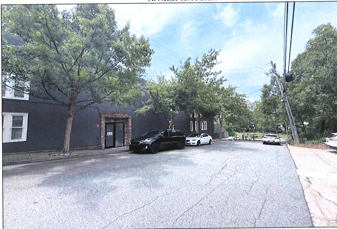
Photograph 10. View toward collocation from Resource 249854, camera facing southwest. A. Nestor 05/15/2025.
