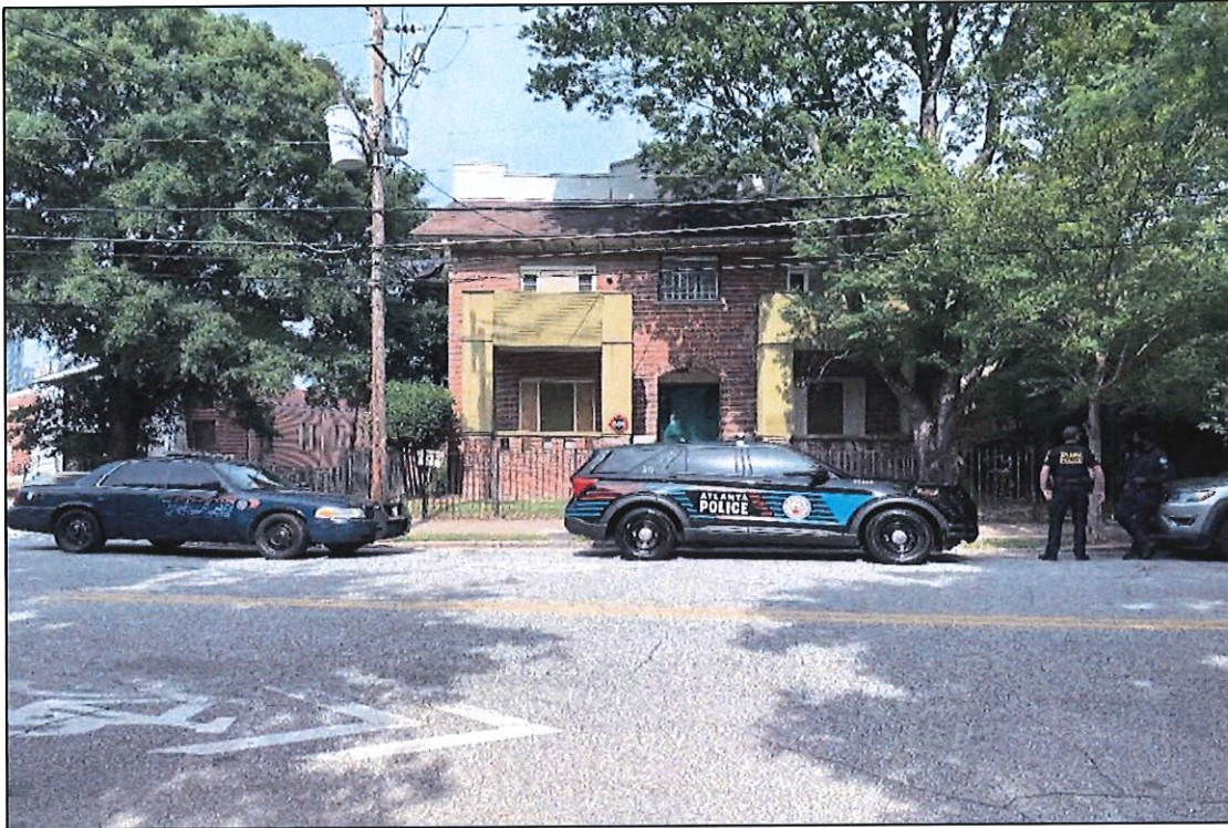
Photograph 77. Overview of Resource 274740, camera facing west. A. Nestor 05/16/2025.
