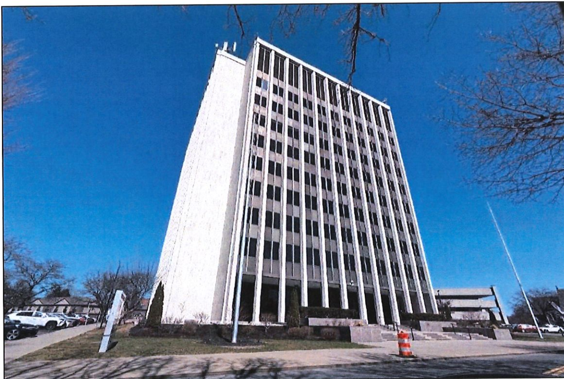
Photograph 4. View toward collocation from Resource 11304.000136, camera facing southwest. A. Nestor 04/01/2025.
