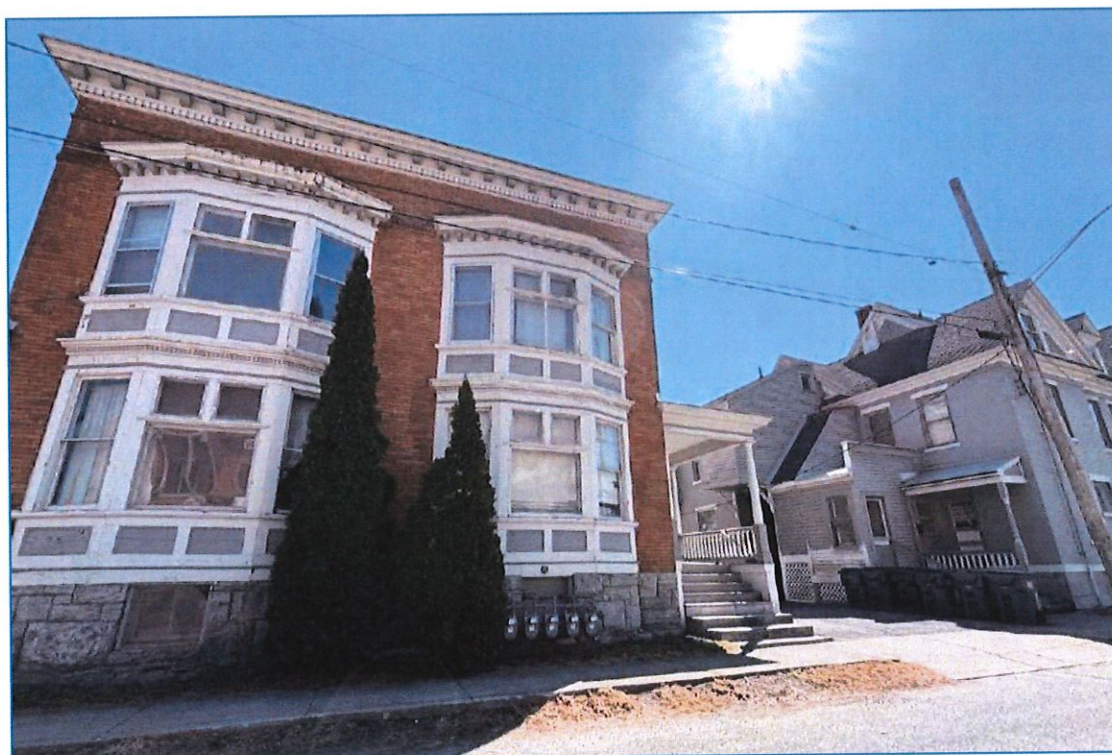
Photograph 96. View toward collocation from Resource 11304.000288, camera facing southeast. A. Nestor 04/01/2025.
