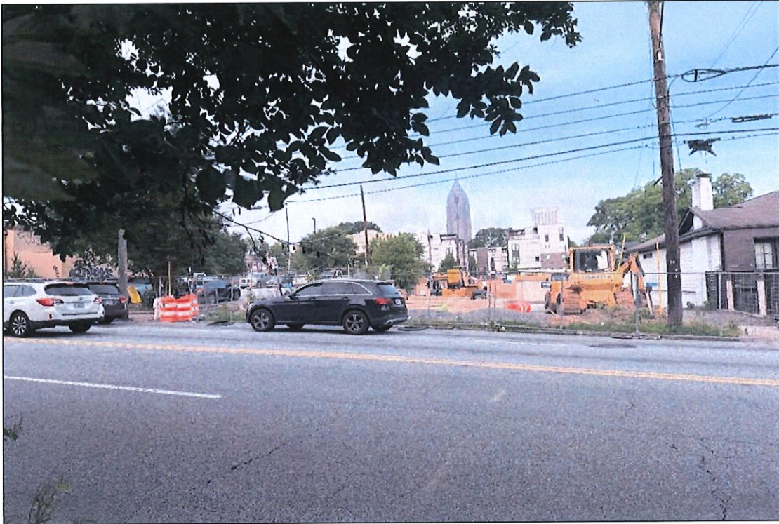
Photograph 33. Overview of Resource 274712, camera facing west. A. Nestor 05/16/2025.
