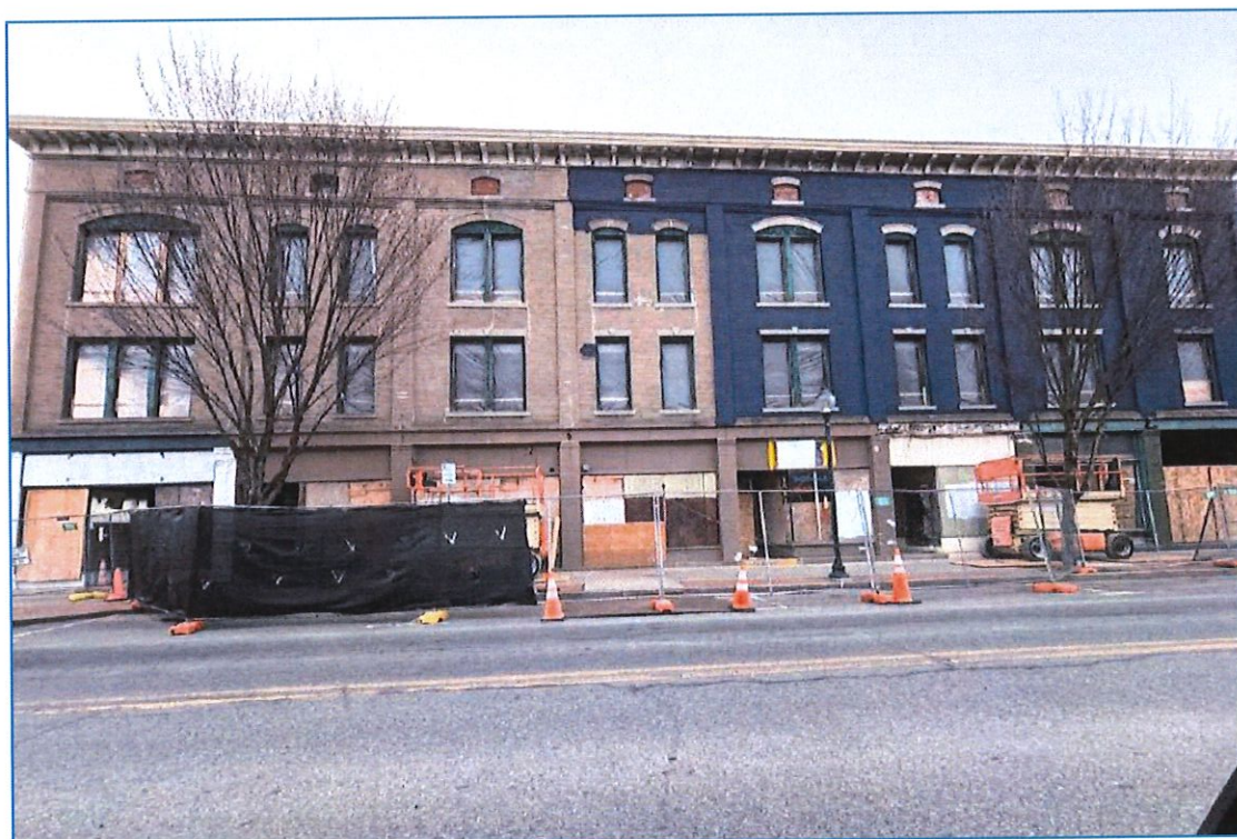
Photograph 60. View toward collocation from Resource 11304.000216, camera facing southeast. A. Nestor 04/02/2025.
