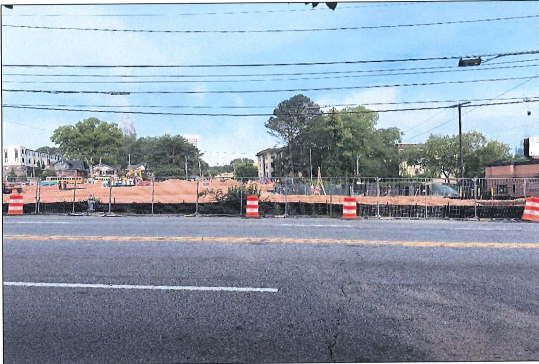
Photograph 29. Overview of Resource 274716, camera facing west. A. Nestor 05/16/2025.
