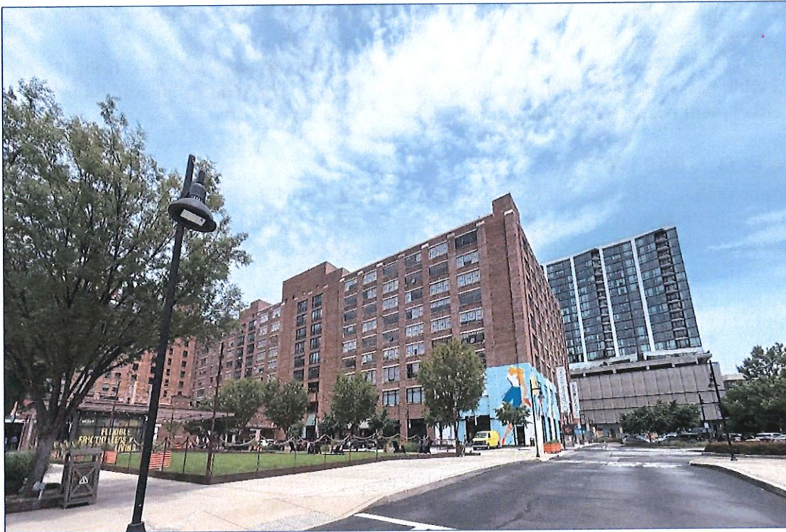
Figure 5. Overview of Project, camera facing northeast. A. Nestor 5/15/2025
