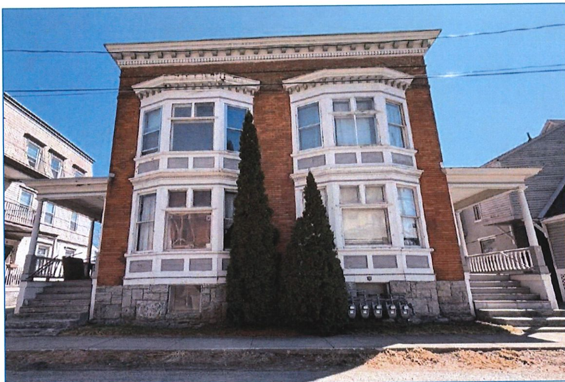
Photograph 95. Overview of Resource 11304.000288, camera facing southeast. A. Nestor 04/01/2025.
