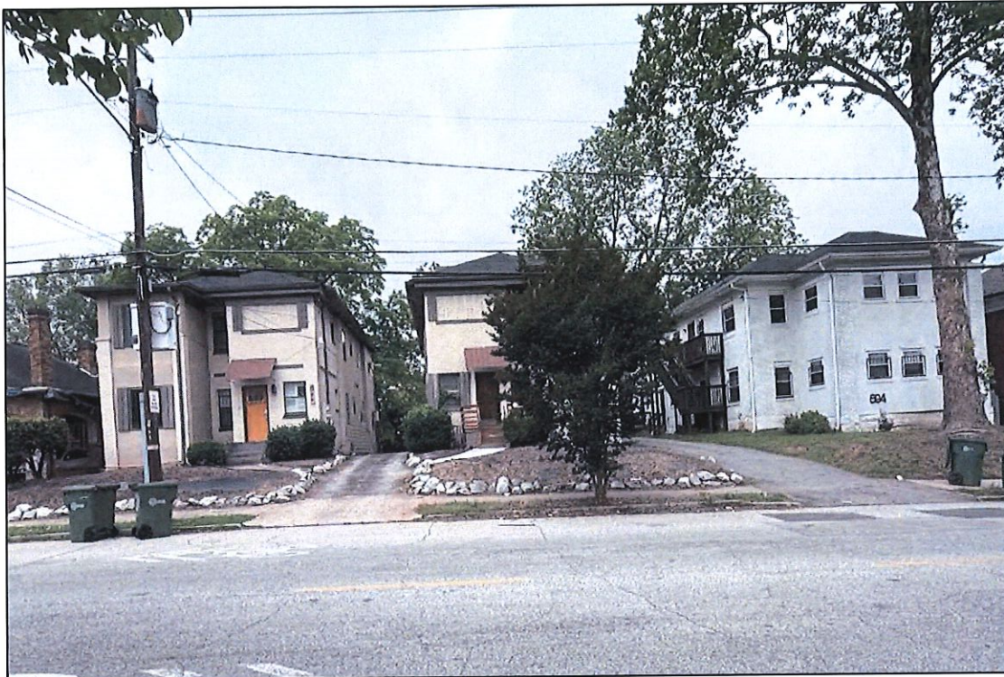
Photograph 53. Overview of Resource 274744, camera facing west. A. Nestor 05/16/2025.
