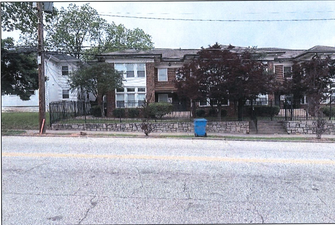
Photograph 49. Overview of Resource 274746, camera facing west. A. Nestor 05/16/2025.
