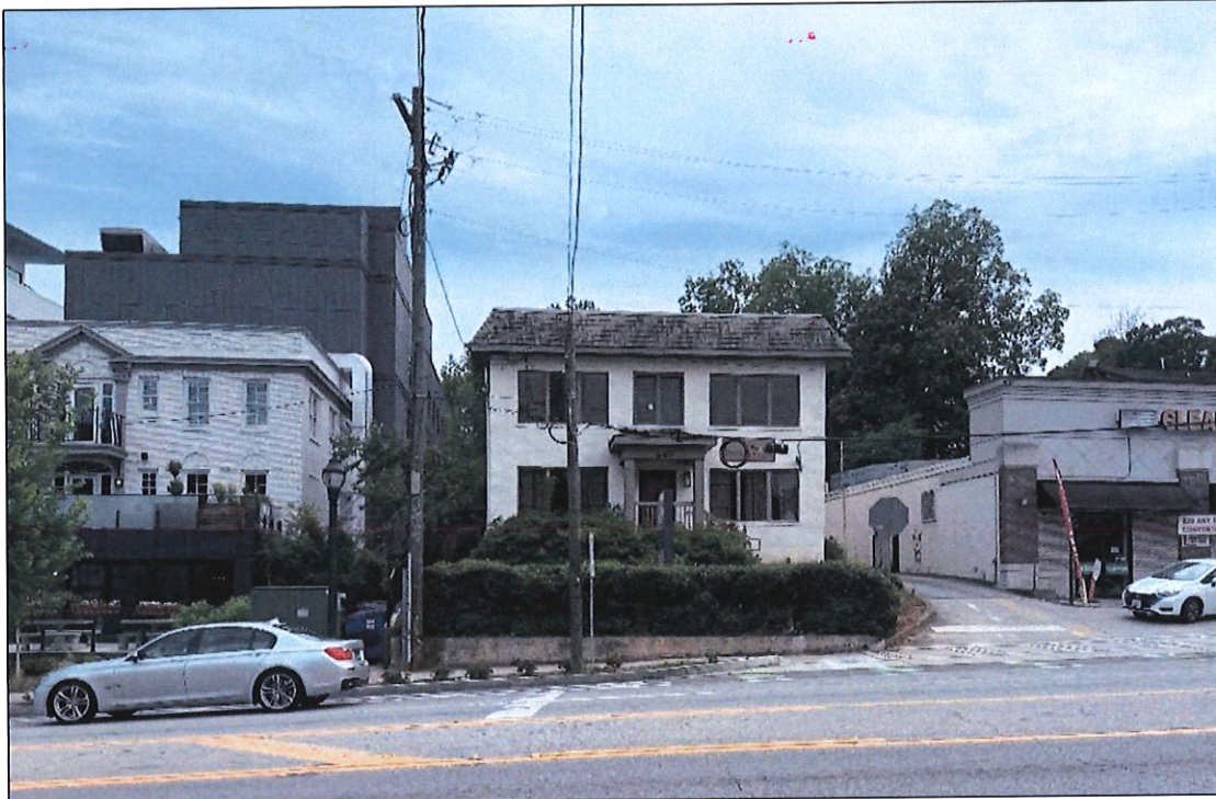
Photograph 21. Overview of Resource 274721, camera facing southeast. A. Nestor 05/15/2025.
