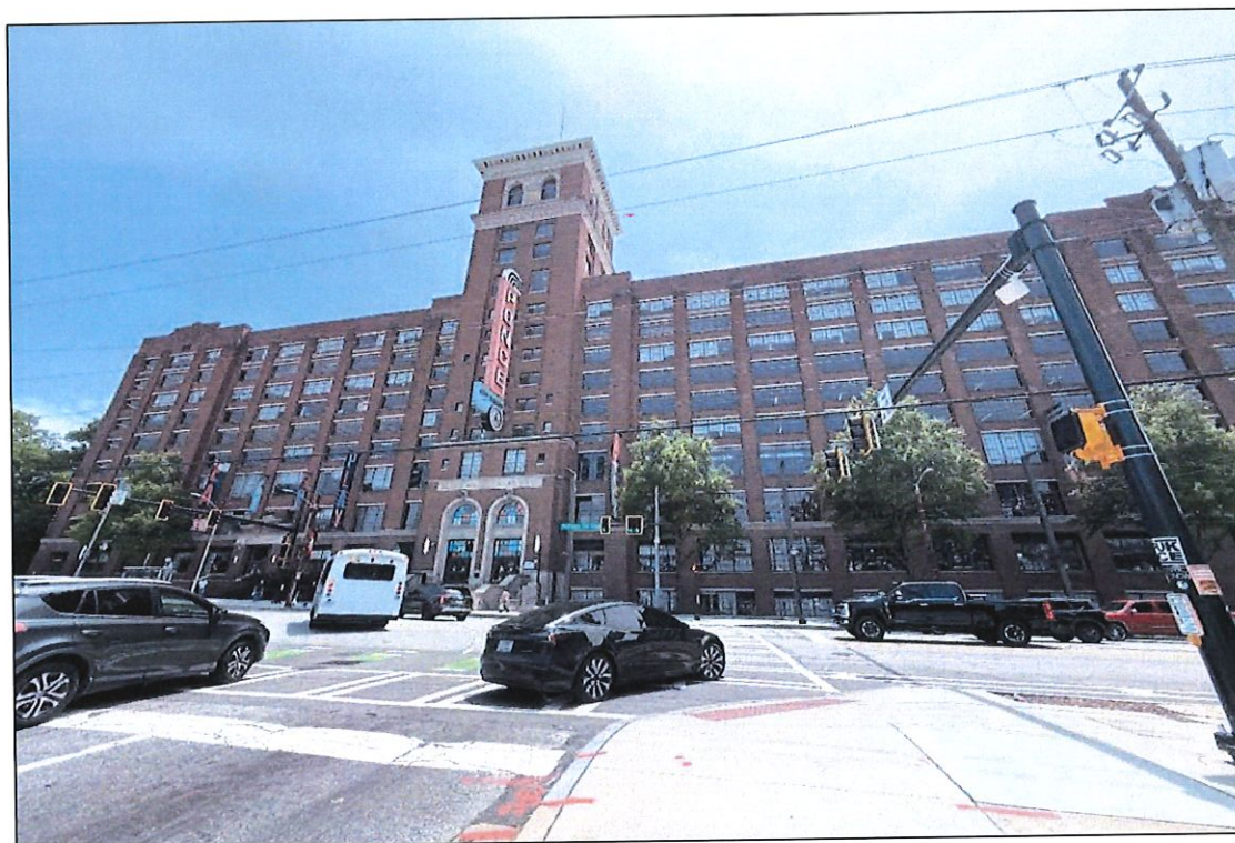
Photograph 2. View toward collocation from Resource 286416, camera facing southwest. A. Nestor 05/15/2025
