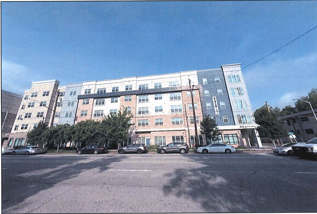
Photograph 85. Overview of Resource 274634, camera facing west. A. Nestor 05/16/2025.
