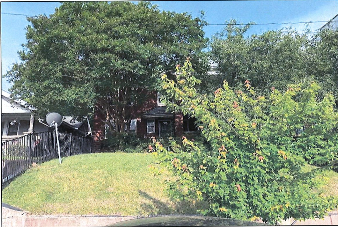
Photograph 81. Overview of Resource 274689 camera facing west. A. Nestor 05/16/2025.
