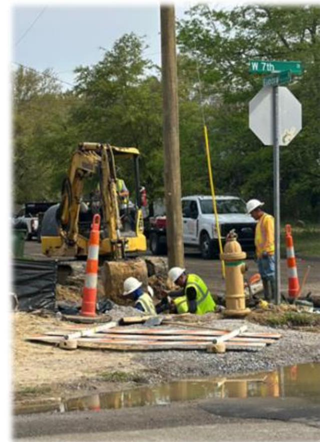
New Utility Lines at W 7 th & Eupora
