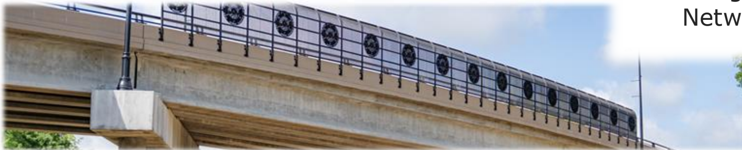
Hall Avenue Overpass
