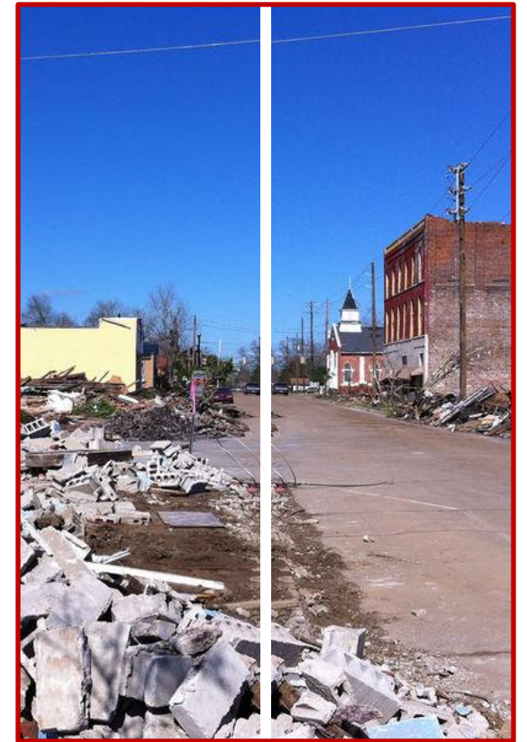
Mobile Street after 2013 Tornado
