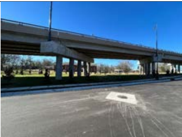
Hall Avenue Over-Pass
