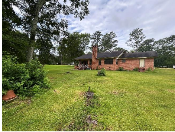
Rear View of Improvements
