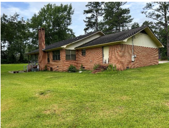
View of improvements from TCE
