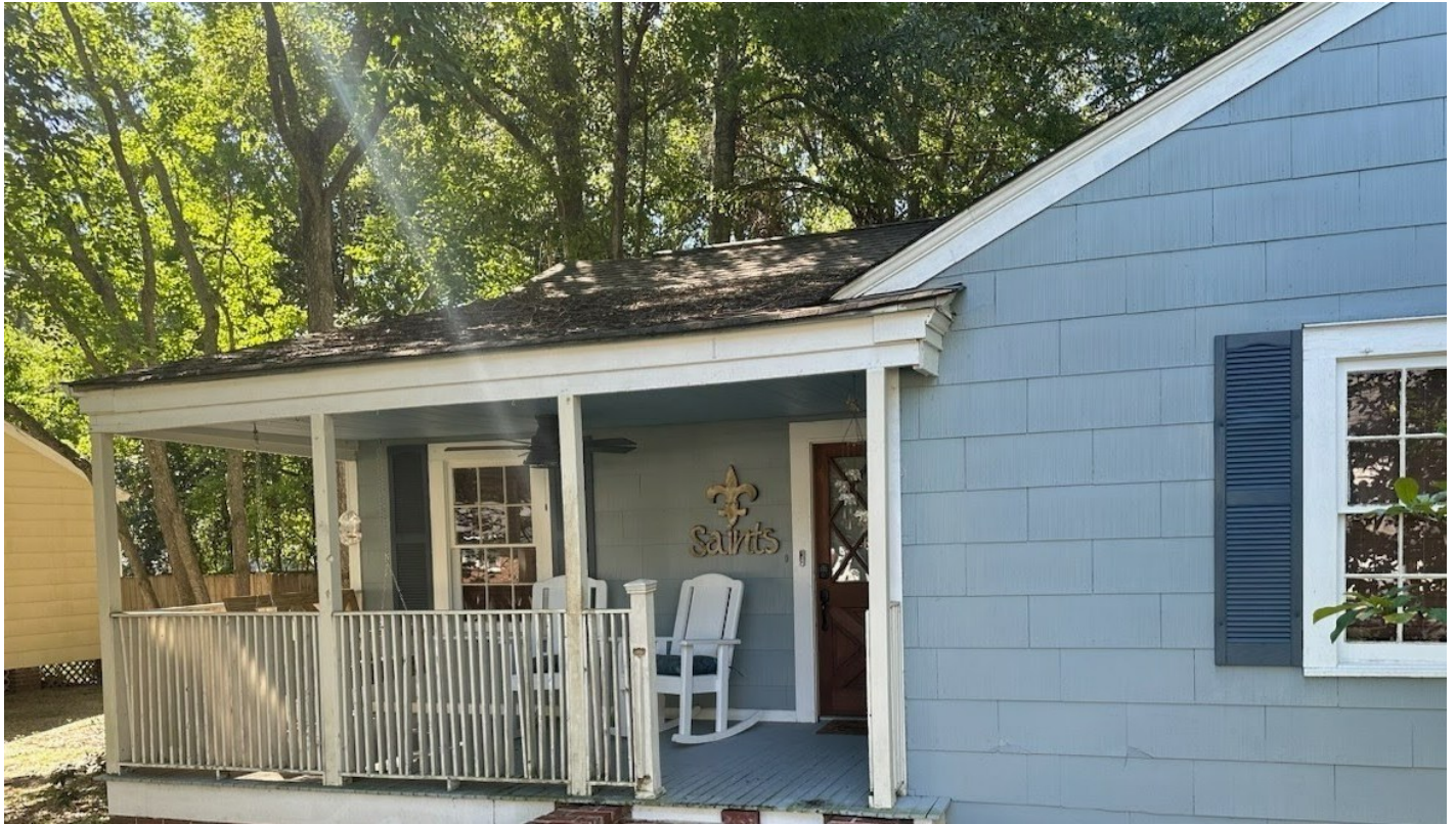
Views of previous porch railing and newly replaced/modified
