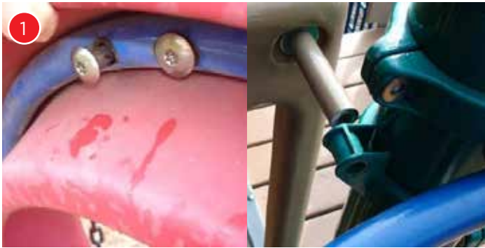
This bolt is loose and should be tightened or replaced.
