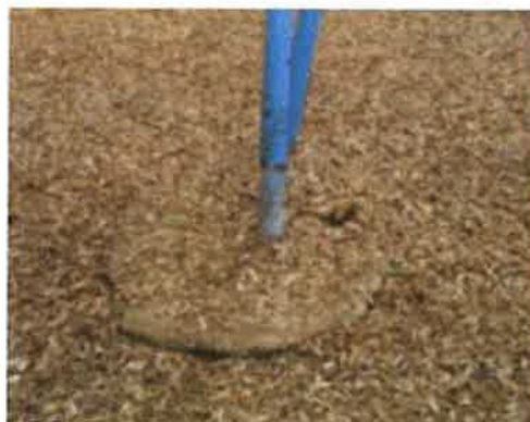
Exposed concrete footing (others)
