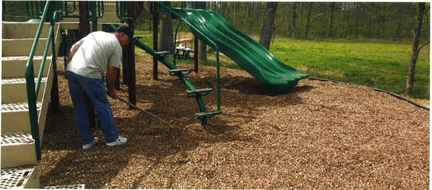
Raking loose-fill engineered wood fiber material
