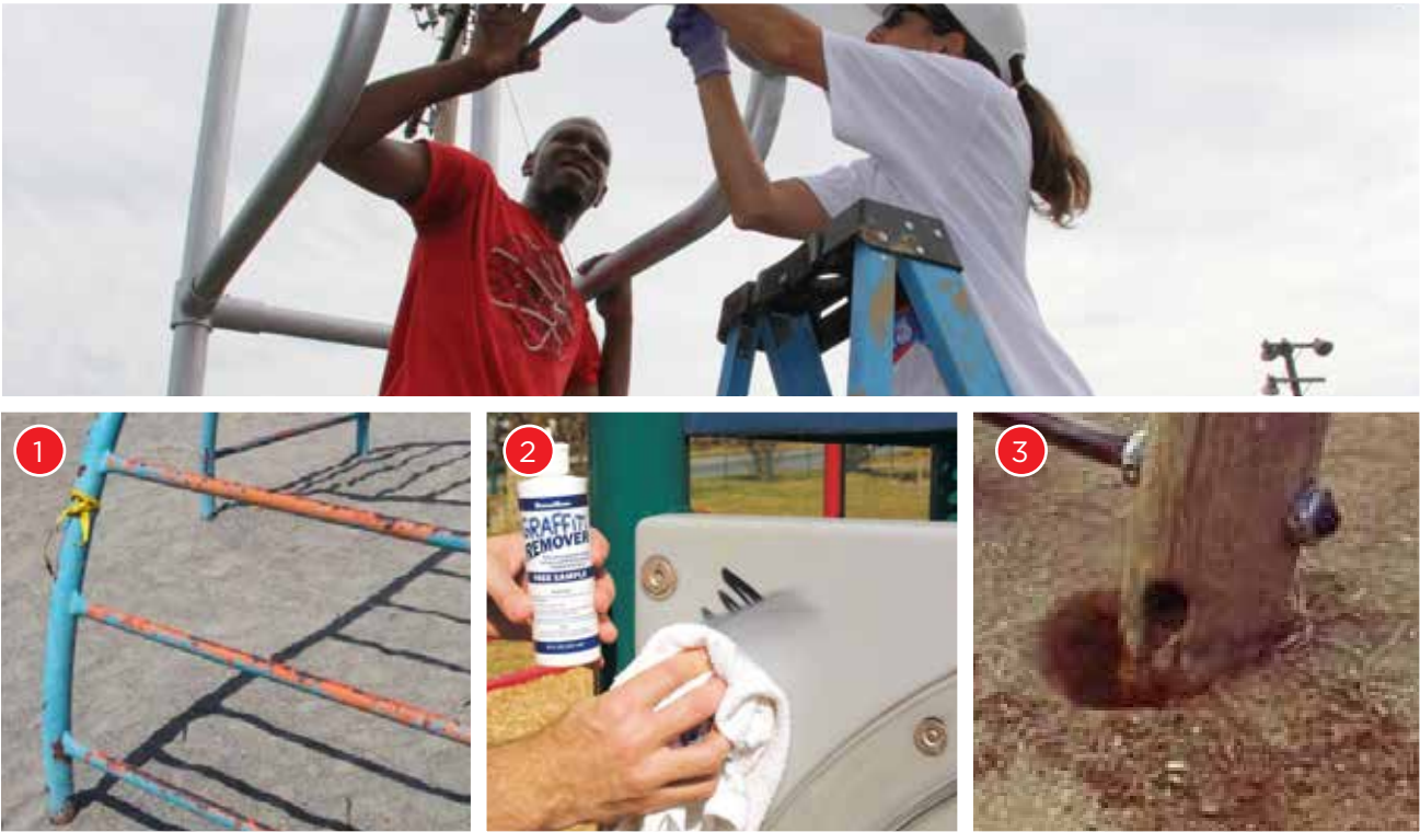
Chipped paint on this equipment should be addressed and repainted.
