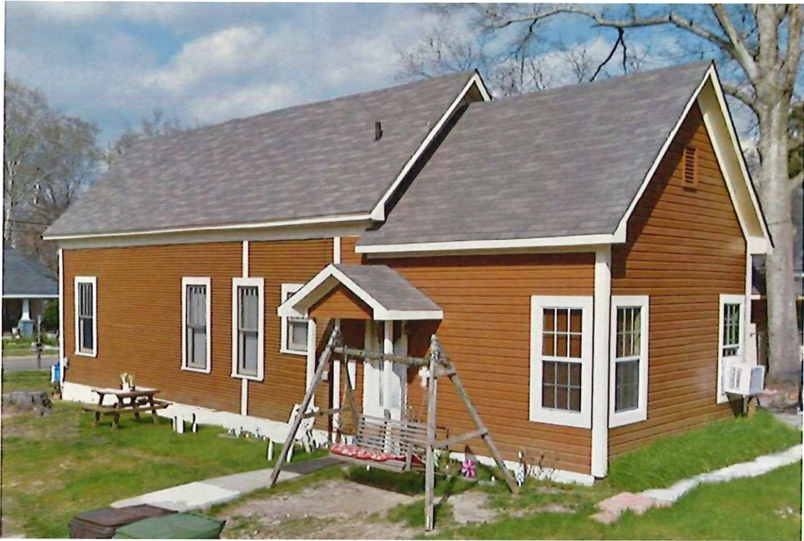
Views of west façade, before and after current work
