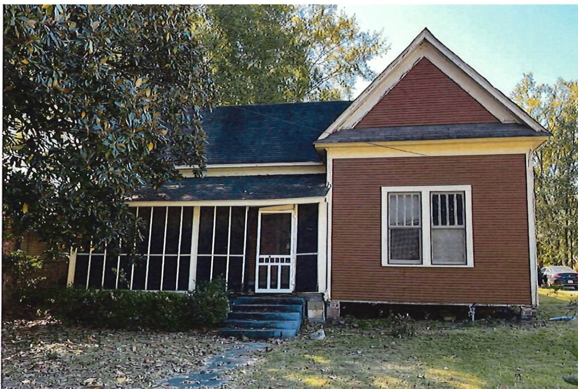
Views of primary façade, before and after window replacement
