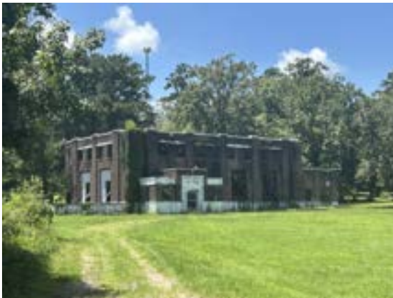
Front of Building
