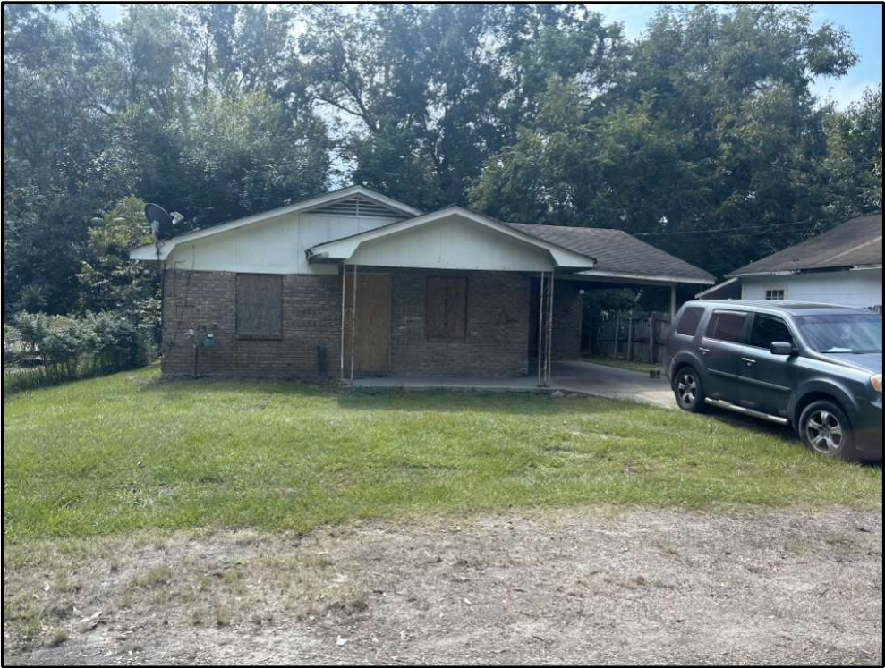
Front of the subject property from Willis Avenue.
