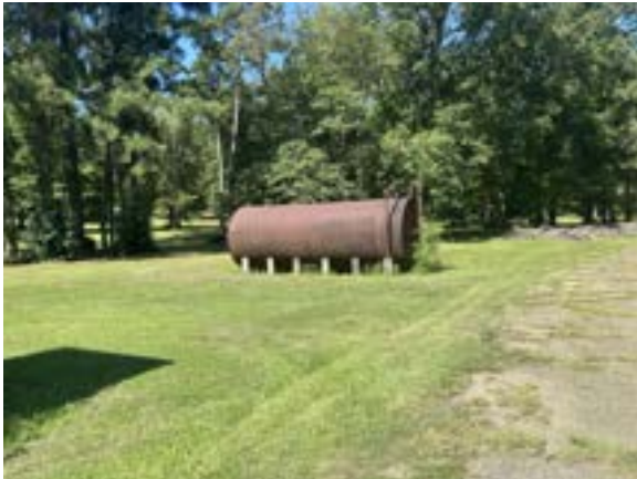
Above-Ground Storage Tank
