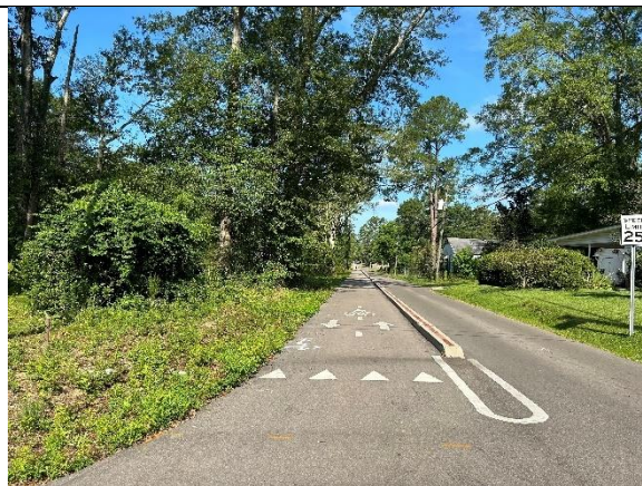
Looking at the property along Camp Street
