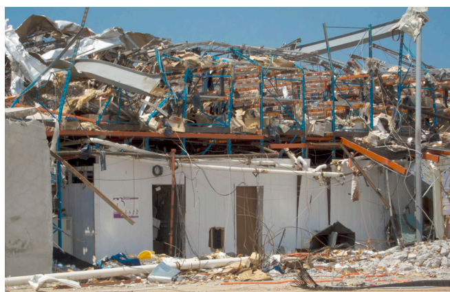
Hackleburg, Alabama, July 19, 2011 -- Almost 90 days after the Wrangler Distribution Center in Hackleburg was destroyed by an EF-5 tornado in Marion County on April 27. Photo by Christopher Mardorf / FEMA. Photo by Christopher Mardorf
