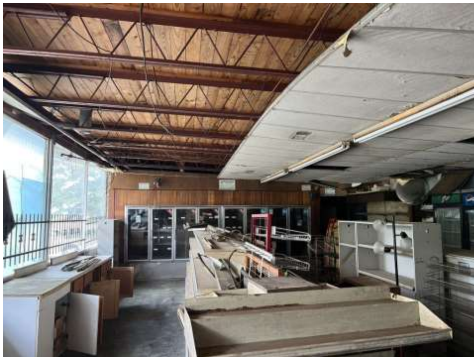
Interior view of retail area
