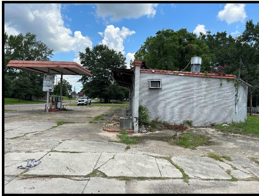
View of the improvements from Southern Avenue
