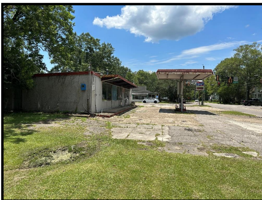
View of the improvements
