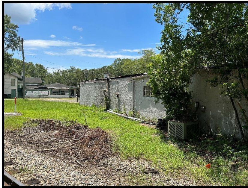
Rear view of the improvements
