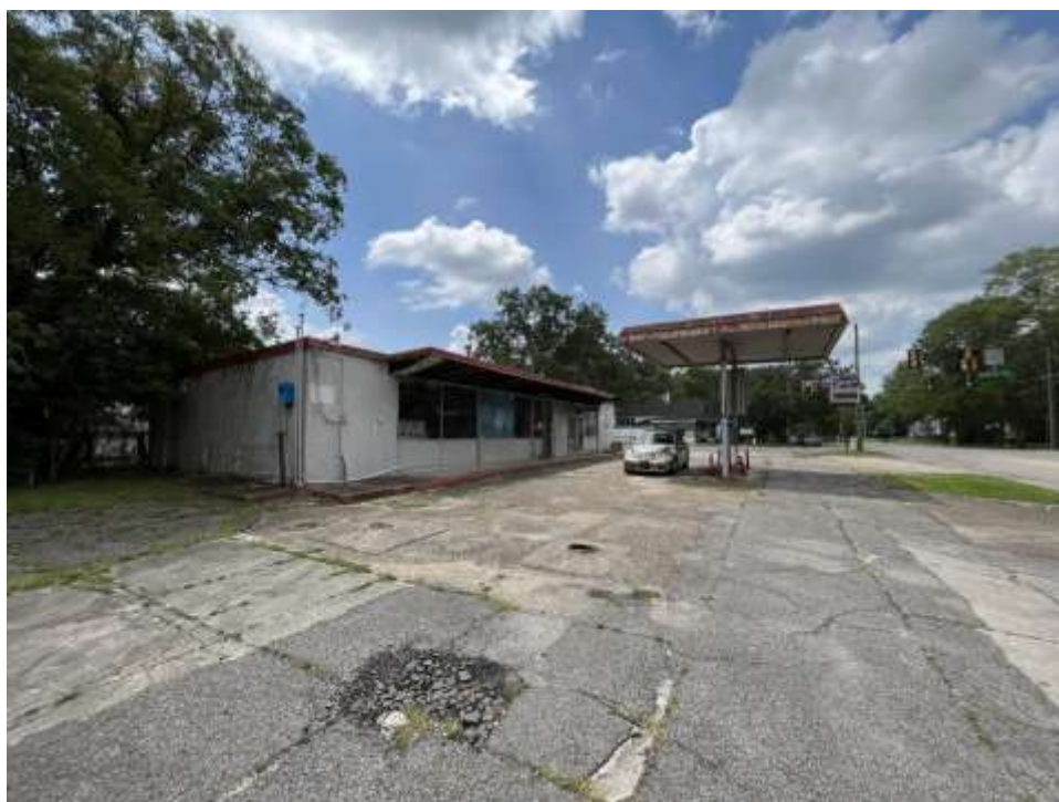
Front view of store
