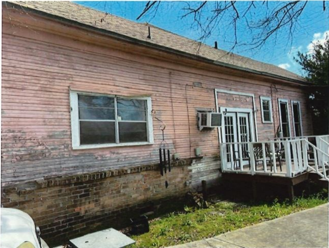
Views of previously replaced windows on rear and west side of house
