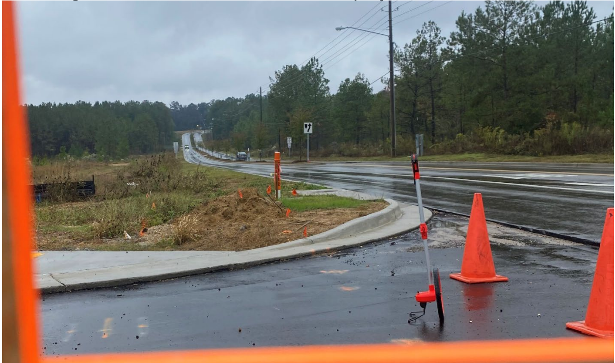
Figure 2: View to the south from Graham Property Drive at Lamar Boulevard
