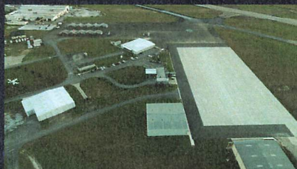
Hattiesburg - Bobby L. Chain Municipal Airport (HBG) Airport Restoration Part 1
