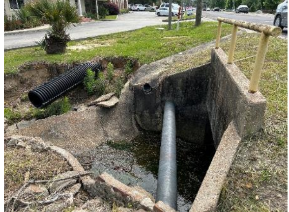
Drainage culvert on the SEC
