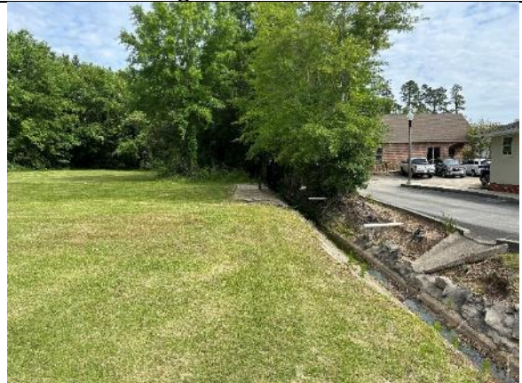
Drainage ditch along the east side of the property
