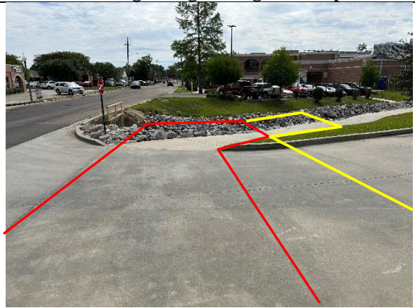
View of permanent and temporary easements located along the access drive and drainage ditch on the east side of the property.
