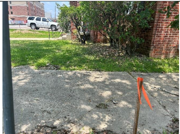
TCE staking along the south property line
