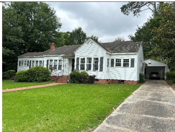
View of the improvements from the proposed acquisition area
