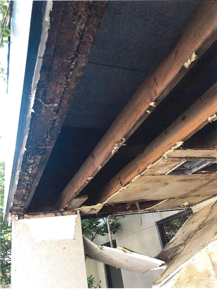
Exterior images of subject building
