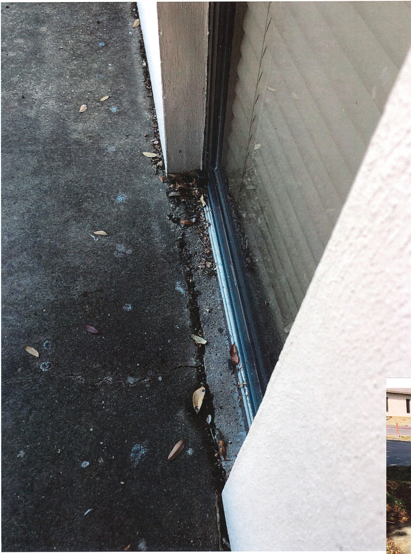
Exterior images of subject building
