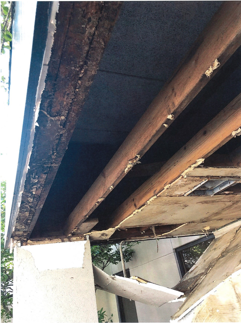
Exterior images of subject building
