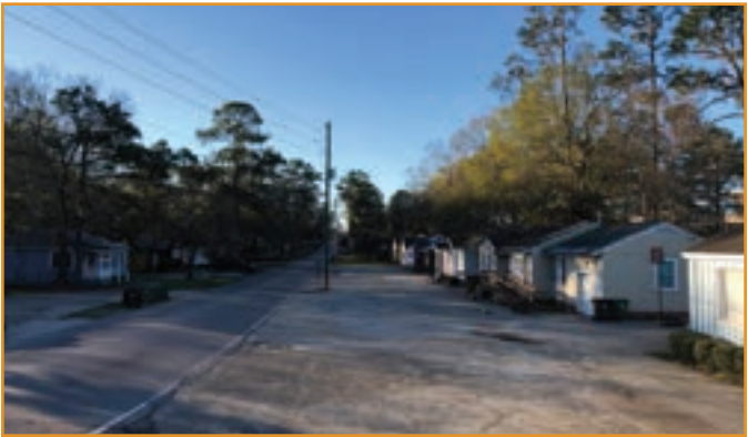
P Continuous driveway frontage and no sidewalks on north end N 25th Ave
