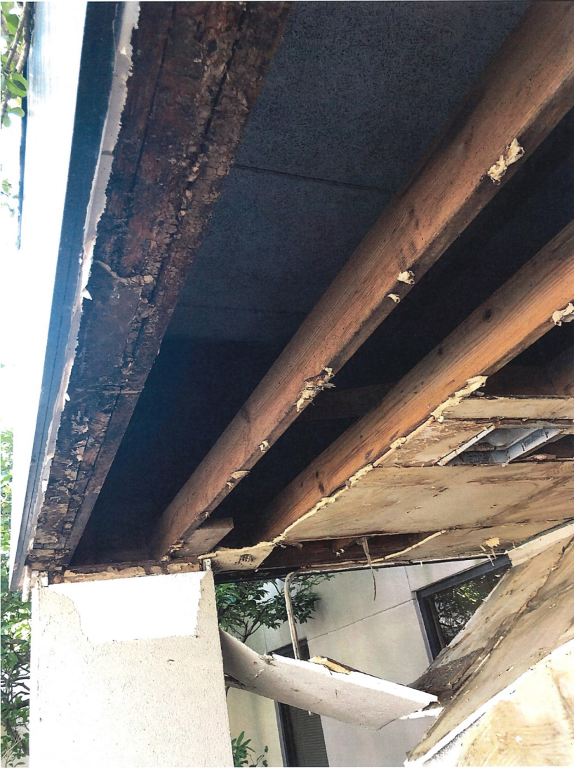
Exterior images of subject building
