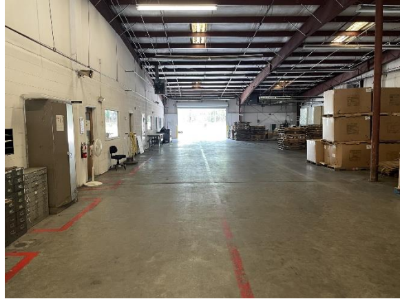
View of rear warehouse (without a/c) Picture taken on October 5, 2022
