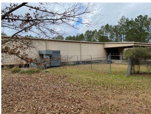
East side of building
