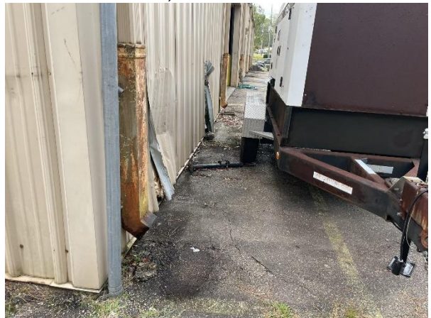
View of northwest exterior Picture taken on October 5, 2022
