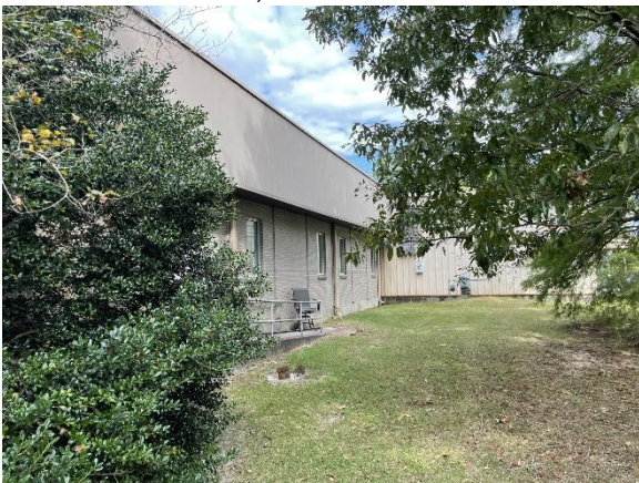
View of west side of office exterior Picture taken on October 5, 2022
