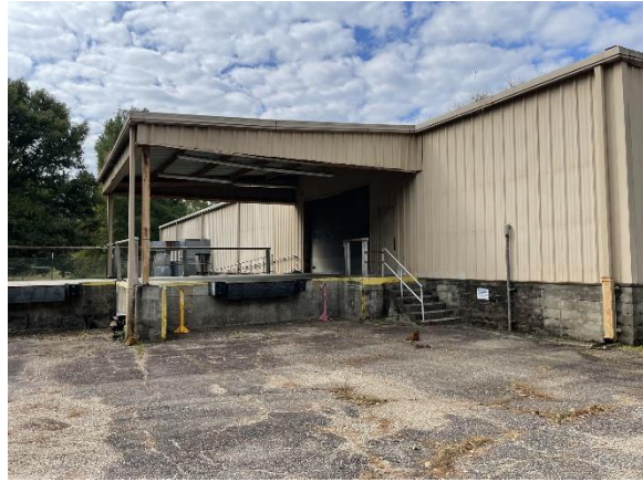
View of loading dock on west side of warehouse Picture taken on October 5, 2022
