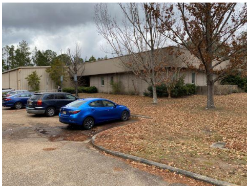
Front of building
