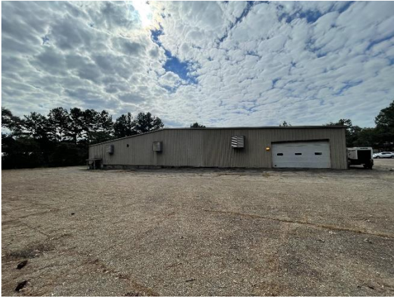
View of north side (rear) of warehouse area Picture taken on October 5, 2022
