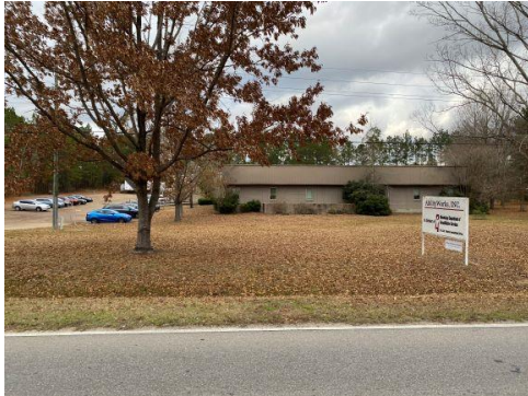
Front of building
