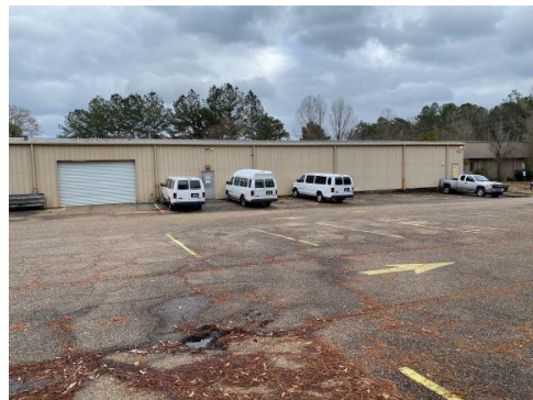
West side of building
