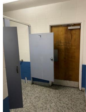
Restroom in warehouse area
