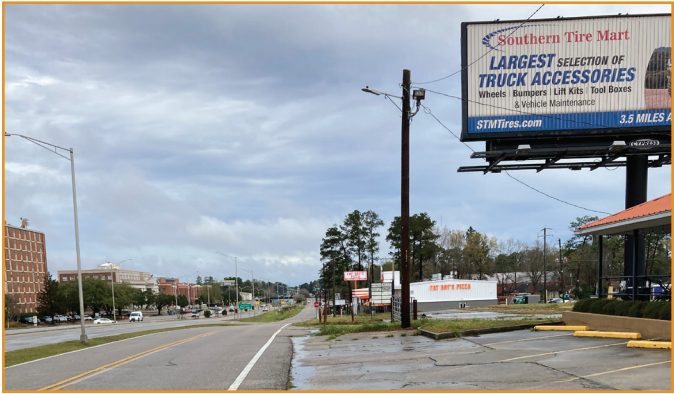
A No continuous curb or sidewalk on N 26th Ave.
