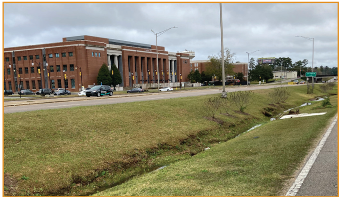
E Deep roadside ditch between Hwy 49 and N 26th Ave.
