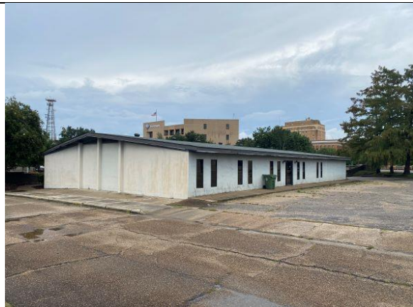
View of the building from Ferguson Street
