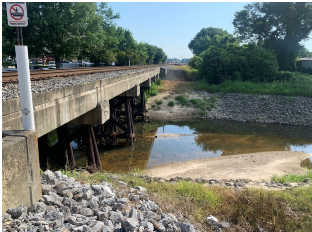
EXISTING VIEW – GORDON'S CREEK View looking North
