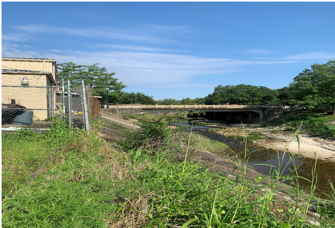
EXISTING VIEW – GORDON'S CREEK View looking West
