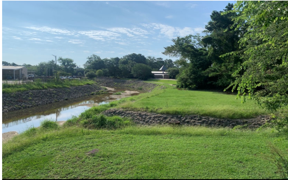
EXISTING VIEW – GORDON'S CREEK View looking West
