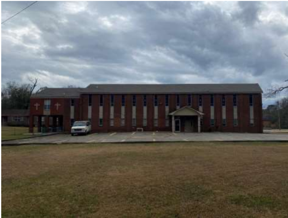
Front view of the church from Martin Luther King Avenue.
