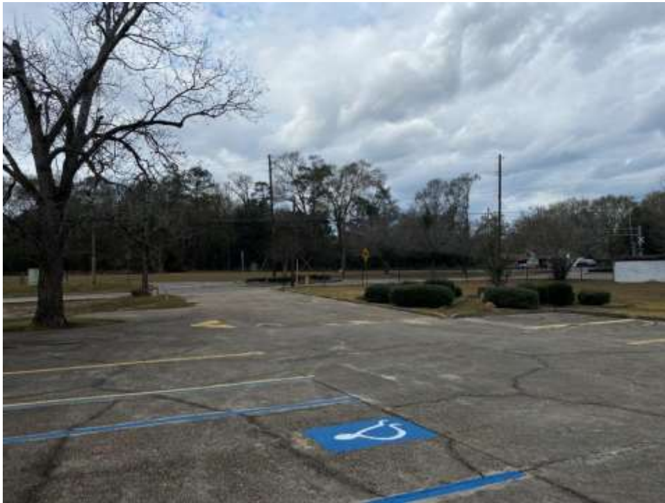
Additional view of the parking lot improvements located outside the proposed acquisition area.
