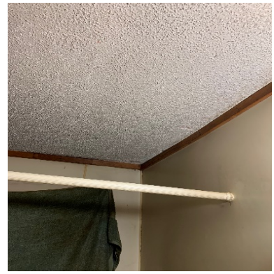
700-AS-03 Ceiling/ Bathroom
