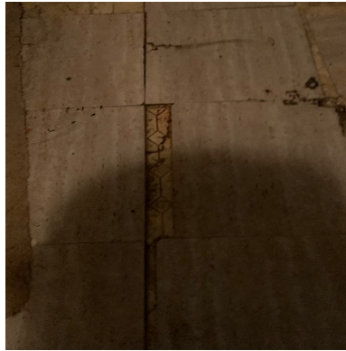
700-AS-05 Linoleum Flooring (Underneath Grey VCT)/ Kitchen
