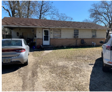
110-AS-02 Transite Siding/Exterior
