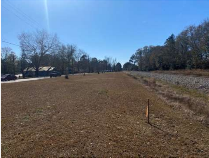
View of "Parcel B" within the proposed right of way.
