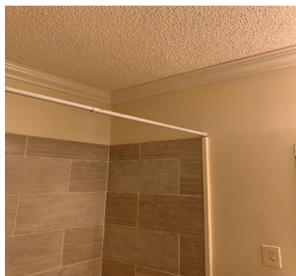
701-AS-02 Ceiling/ Bathroom
