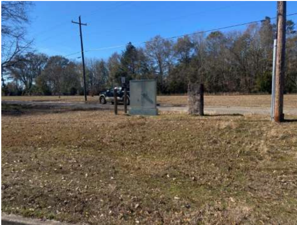
View of the utility related structures located in the proposed acquisition area.
