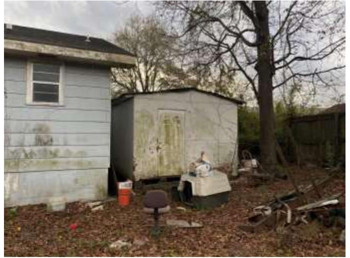
Additional view of the rear of the house and the storage building on the property.
