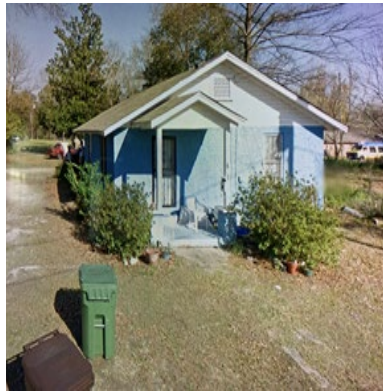
700-AS-02 Transite Siding/ Exterior
