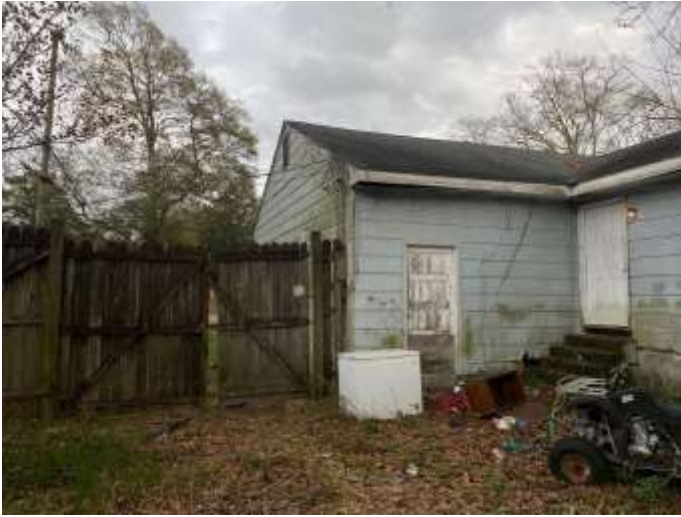
View of the rear of the house.
