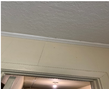
110-AS-07 Ceiling/ Kitchen
