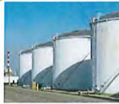
Bulk Storage Facilities
