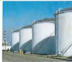
Bulk Storage Facilities
