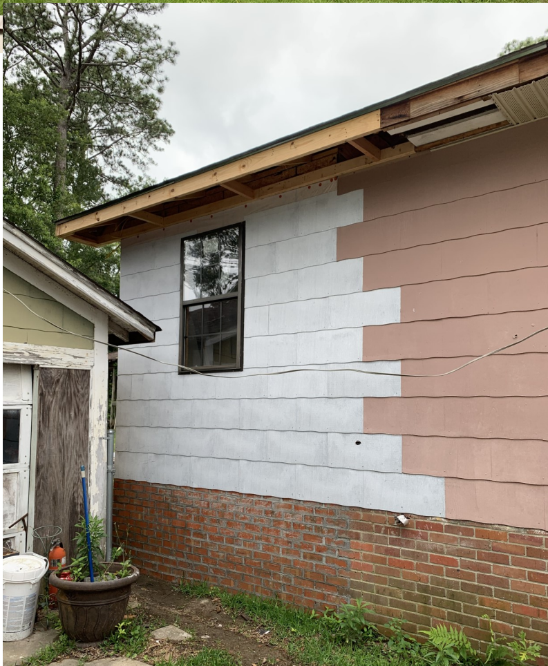
Project area from east (driveway area)
