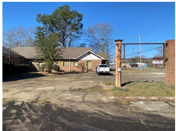
Additional view of parking area in front of the building.
