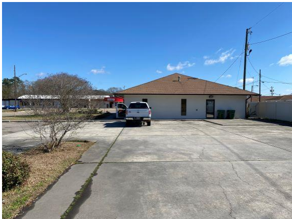
Parking lot located along W. Florence Street
