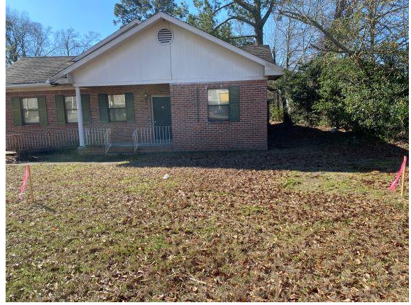
Looking towards the building at the proposed r.o.w.
