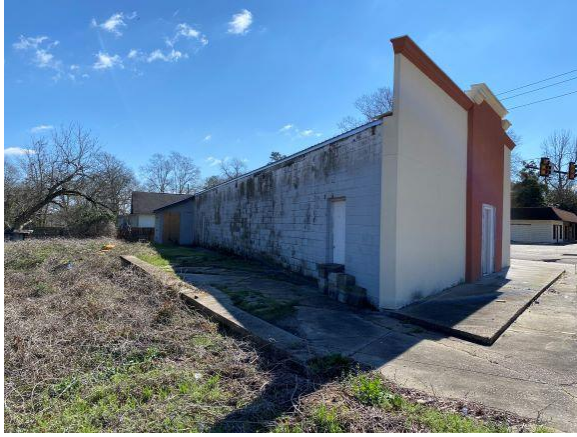
North side of the building from Main Street
