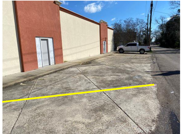
Looking east along E. 7 th Street at the front of the building
