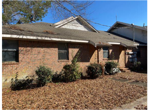
Rear of the building
