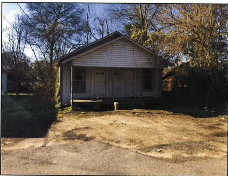
Front of the subject property from Willis Avenue.
