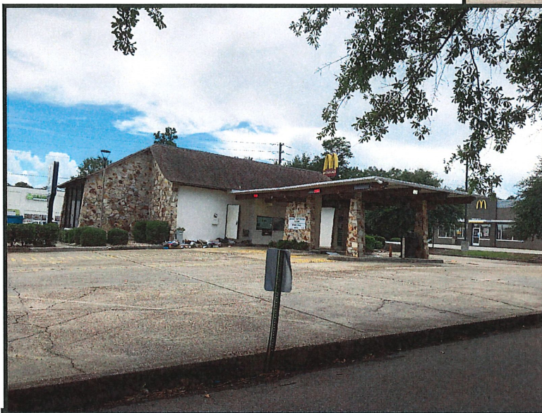
REAR OF SITE LOOKING SOUTHWEST
