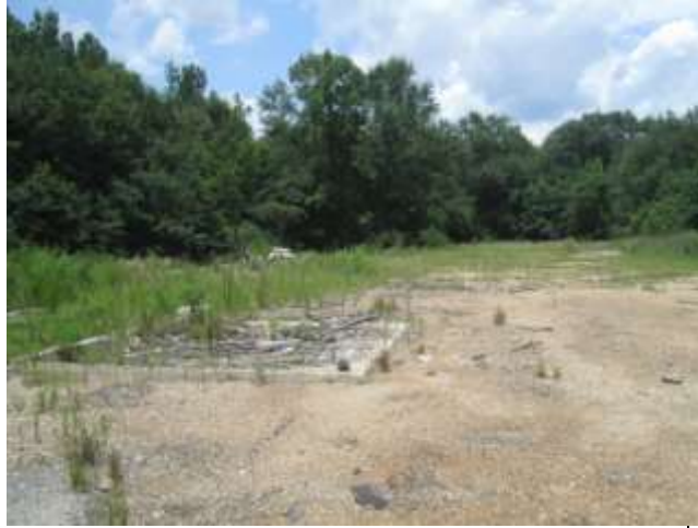
Exterior view of the east side of the building.
