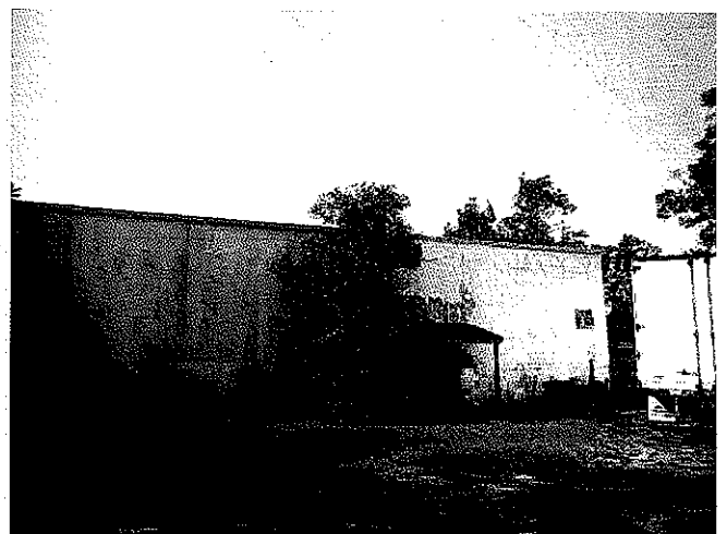
View of northerly side of building
