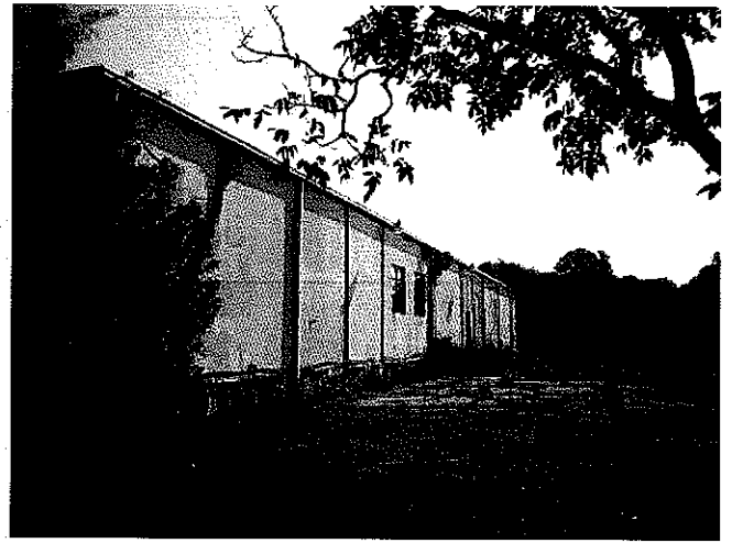
View of southerly side of building
