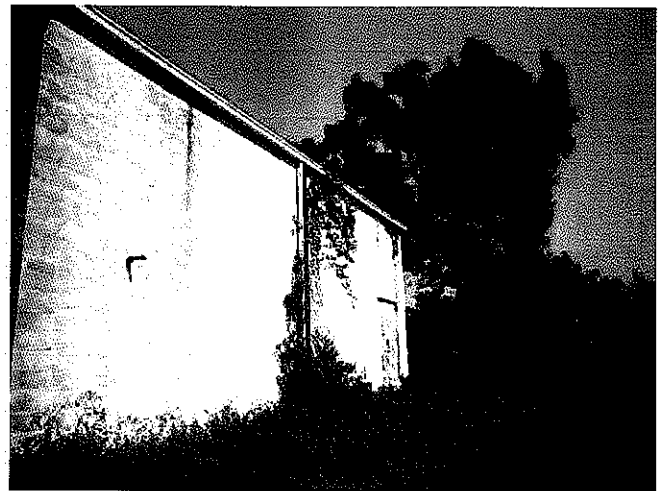
View of easterly side of building
