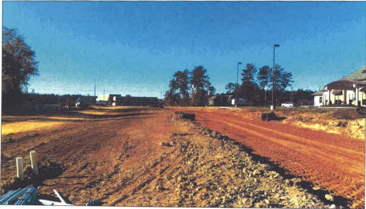
Figure 7 – Engineer Stakes Locations of Light Poles for Electrical Contractor (looking South) (11/22/17)
