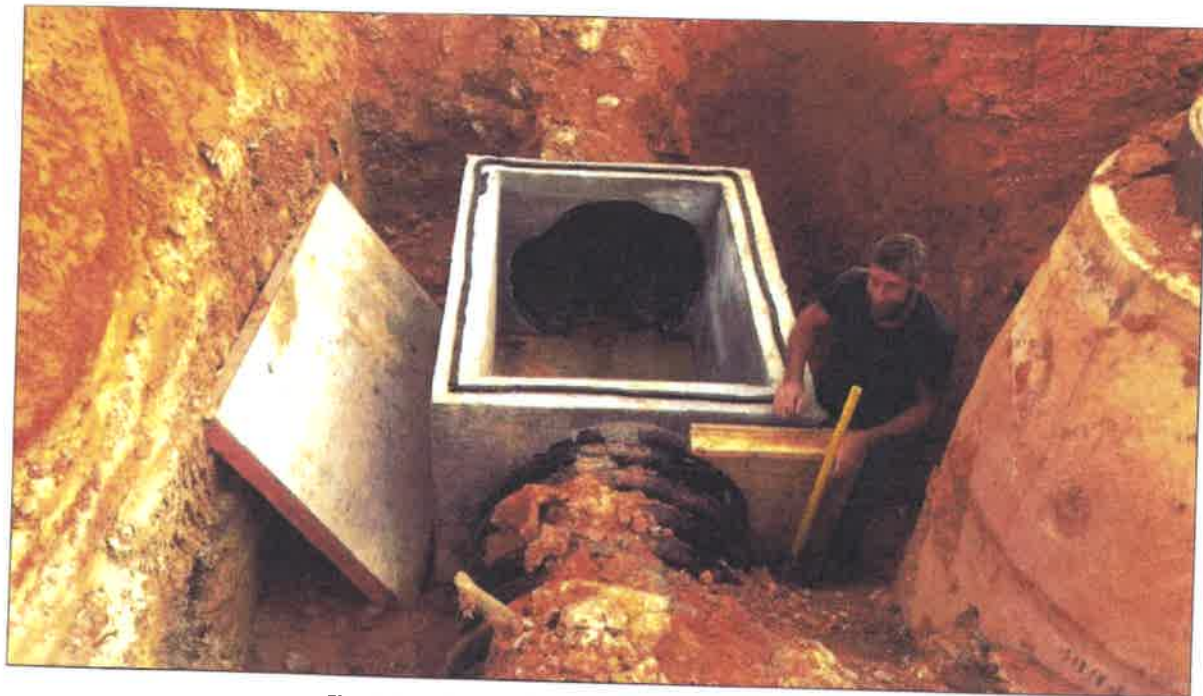
Figure 2 – All Storm Drainage Work Complete (11/6/17)
