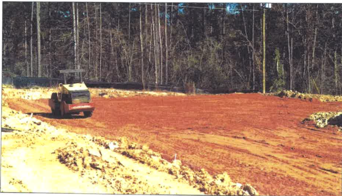
Figure 6 – Borrow Material Placed Over Geogrid in Cul-De-Sac Area (11/21/17)
