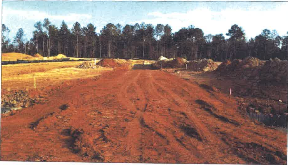
Figure 3 – Subgrade Rough Grading Commences (looking North) (11/17/17)
