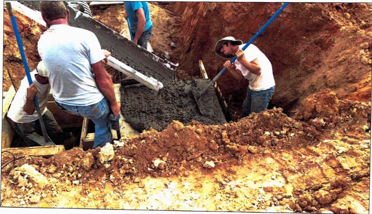
Figure 1 – Pouring Concrete for Inlet 1 (11/3/17)
