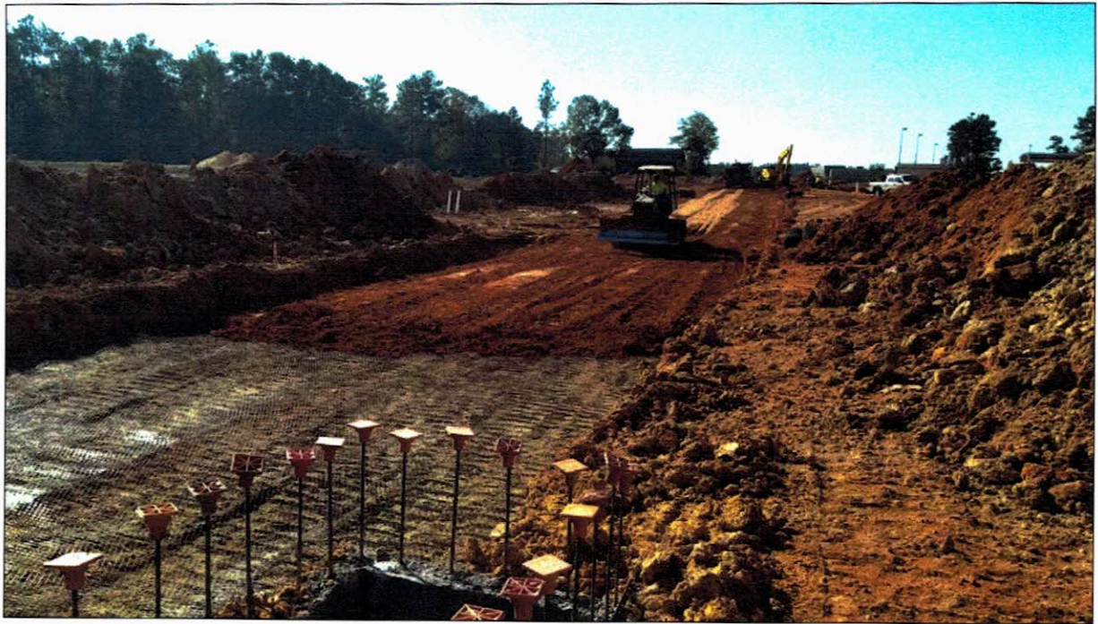
Figure 5 – Unclassified Excavation Being Placed on Geogrid (11/17/17)
