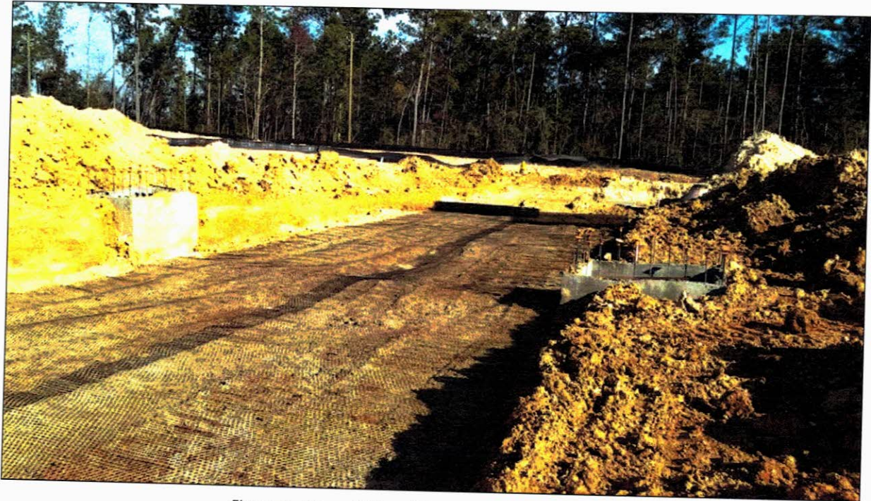
Figure 4 – Geogrid Placed Near Station 8+00 (11/17/17)
