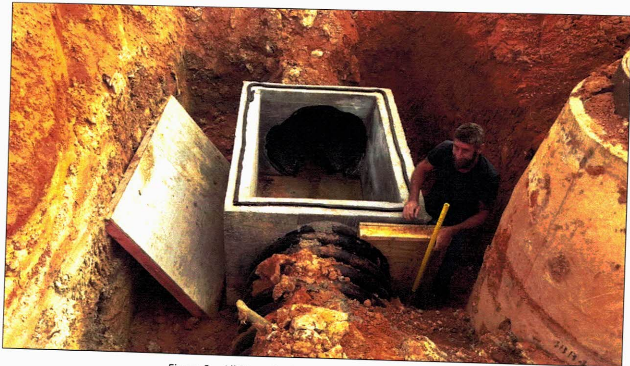
Figure 2 – All Storm Drainage Work Complete (11/6/17)
