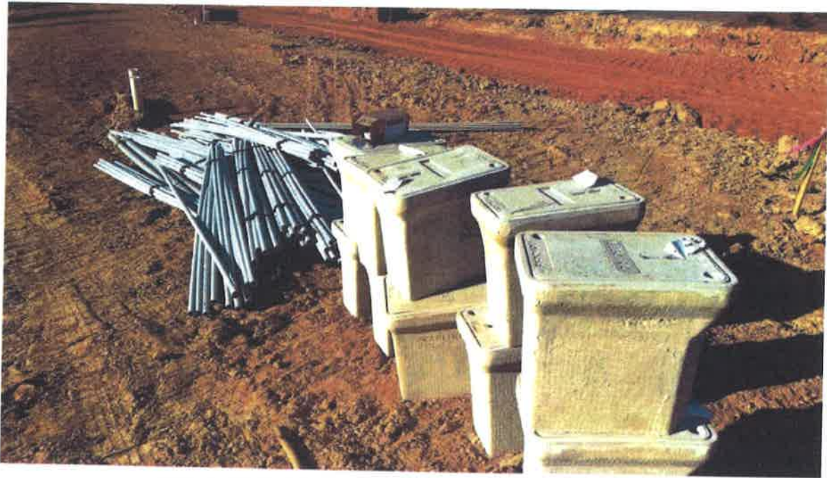
Figure 8 – Electrical Contractor Begins Installation of Conduits (11/28/17)
