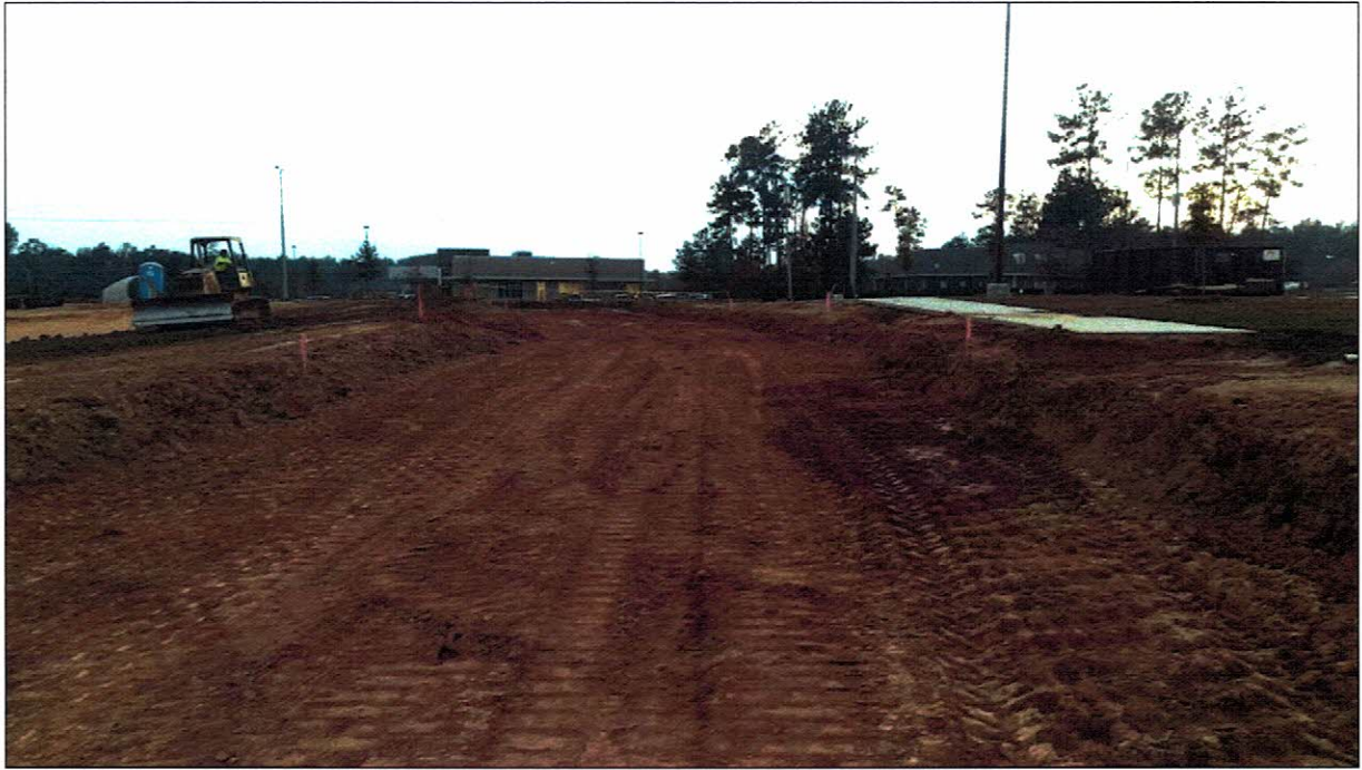
Figure 9 – All Subgrade Rough Grading and Electrical Conduit Installation Complete (11/29/17)
