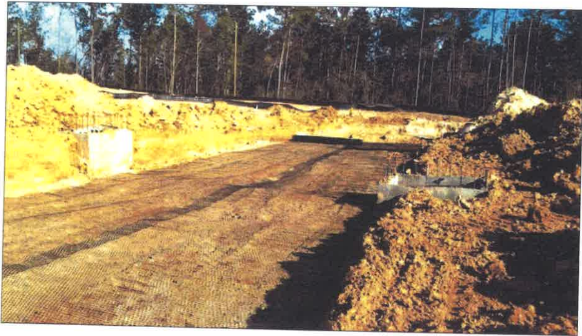
Figure 4 – Geogrid Placed Near Station 8+00 (11/17/17)
