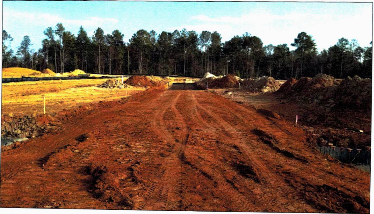
Figure 3 – Subgrade Rough Grading Commences (looking North) (11/17/17)
