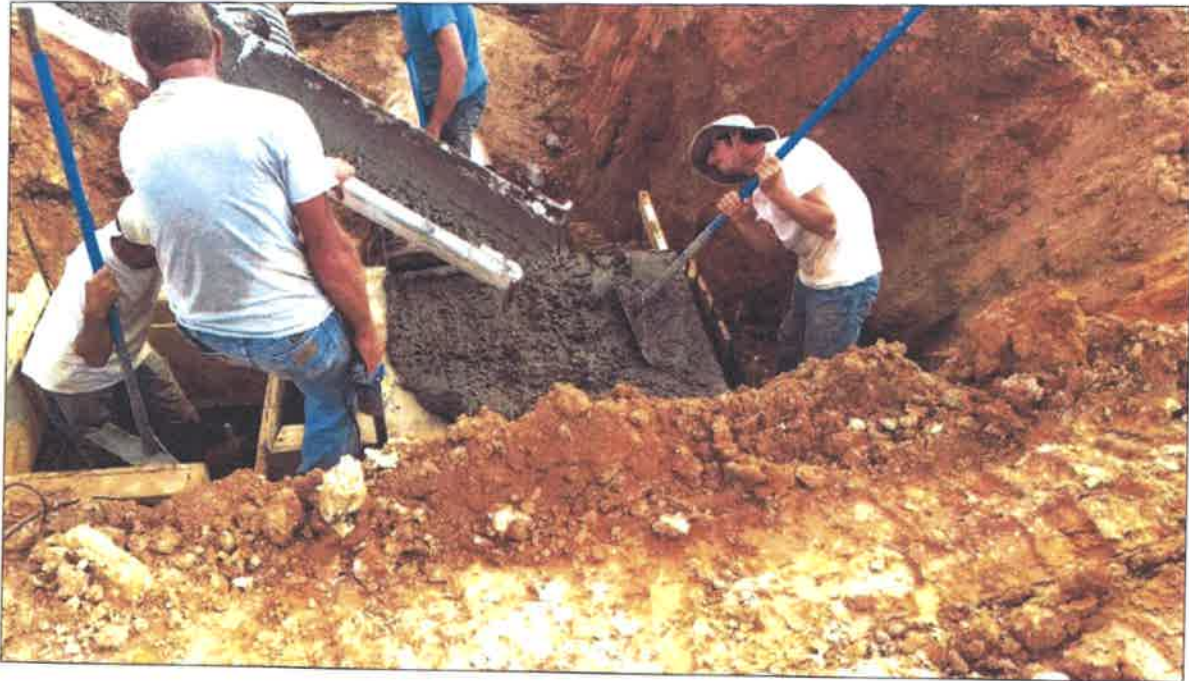
Figure 1 – Pouring Concrete for Inlet 1 (11/3/17)
