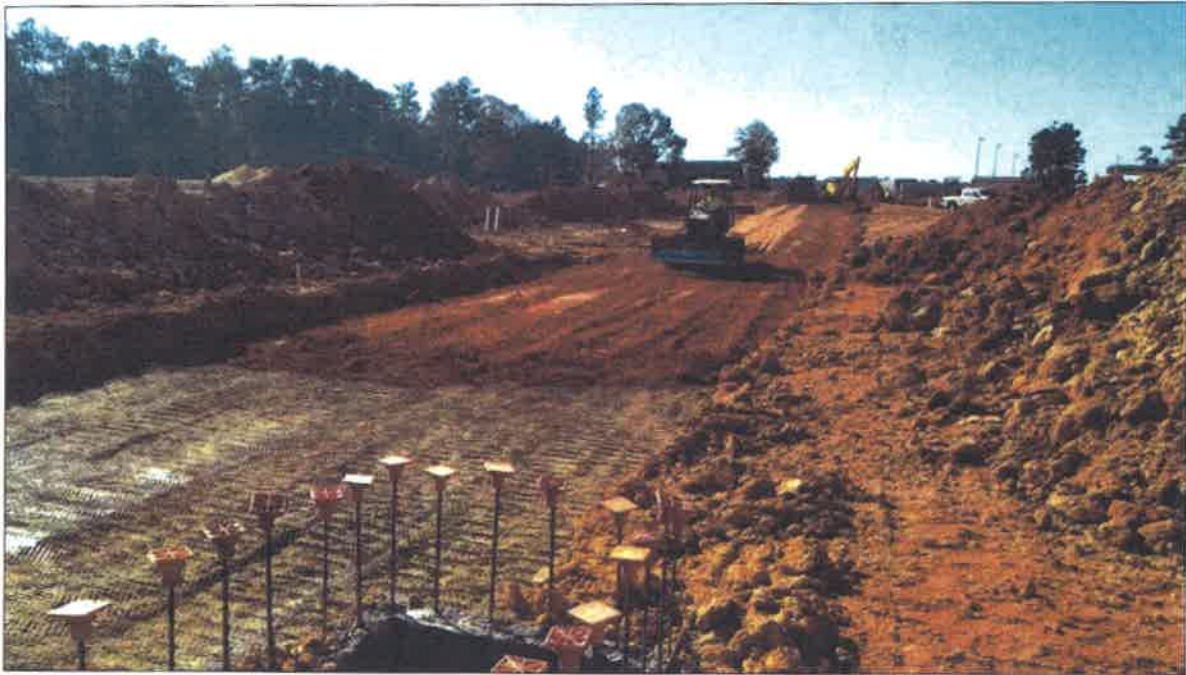
Figure 5 – Unclassified Excavation Being Placed on Geogrid (11/17/17)
