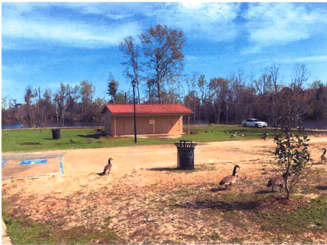
Existing Restroom Facility Duncan Lake Park
