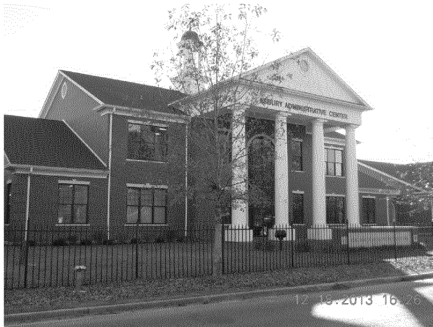
EXISTING VIEW – TUSCAN AVENUE View to the Southwest: Looking at the Asbury Administrative Center College of Osteopathic Medicine: William Carey University
