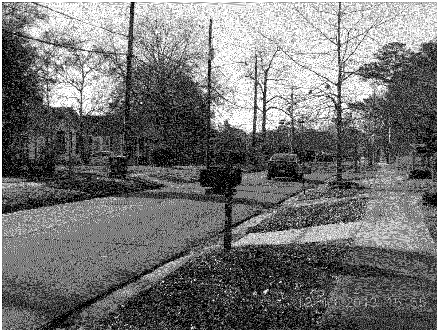
EXISTING VIEW – TUSCAN AVENUE View to the West between Cedar St. and Cherry St.
