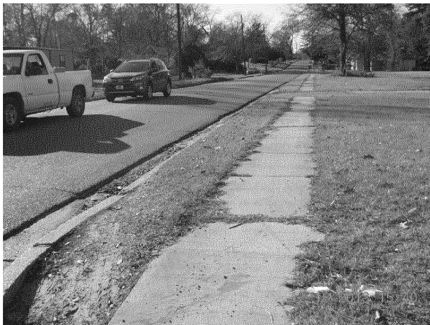
EXISTING VIEW – TUSCAN AVENUE View to the West at Edwards Street
