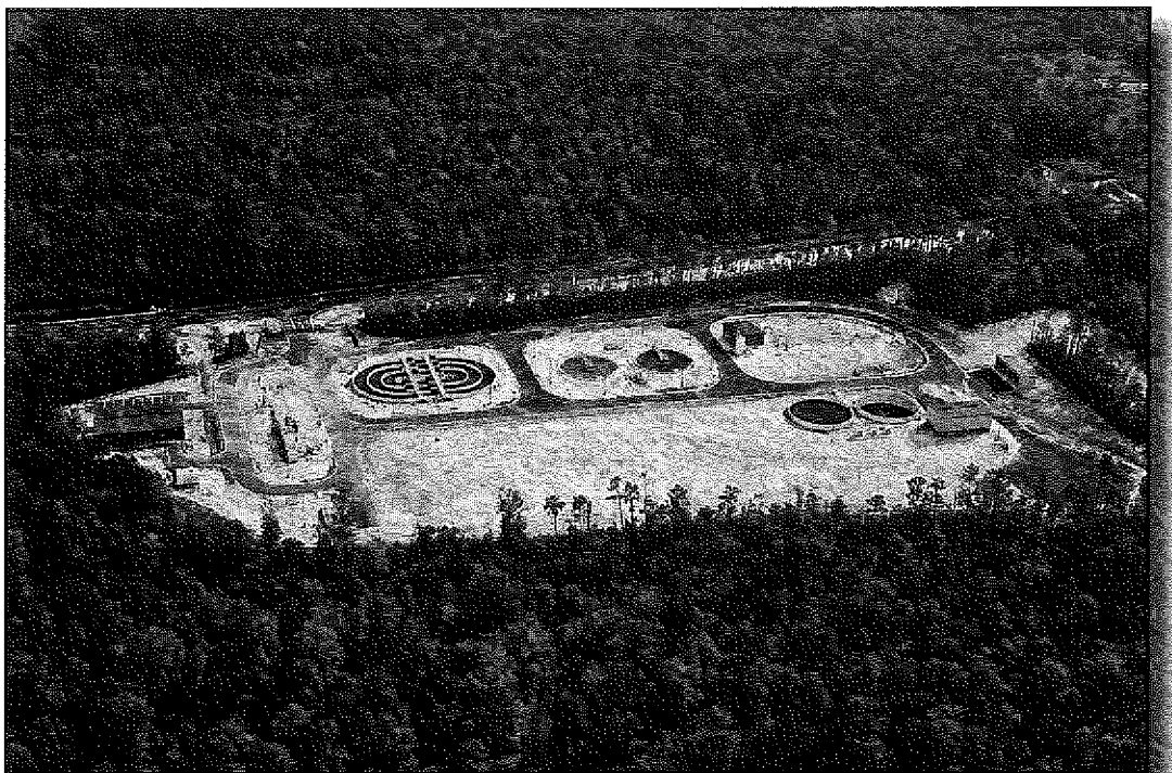
Woolmarket Wastewater Treatment Facility, Woolmarket, MS
