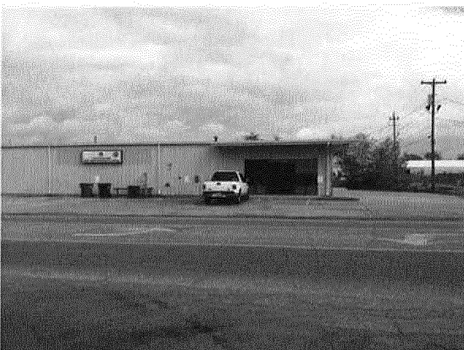
Property to the East
