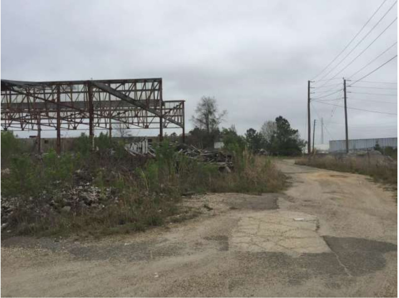
Remnant steel structure and wood floors from former warehouse building on the subject property
