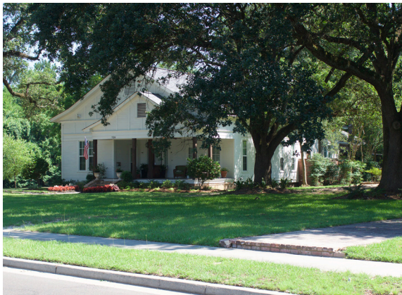
TFR homes in various states of repair.
