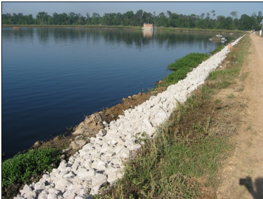
Figure 1-5. View of Riprap Repairs at North Lagoon.
