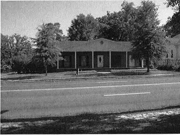
Office Building Directly Across Street (North)
