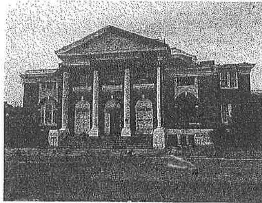
South Side Building C
