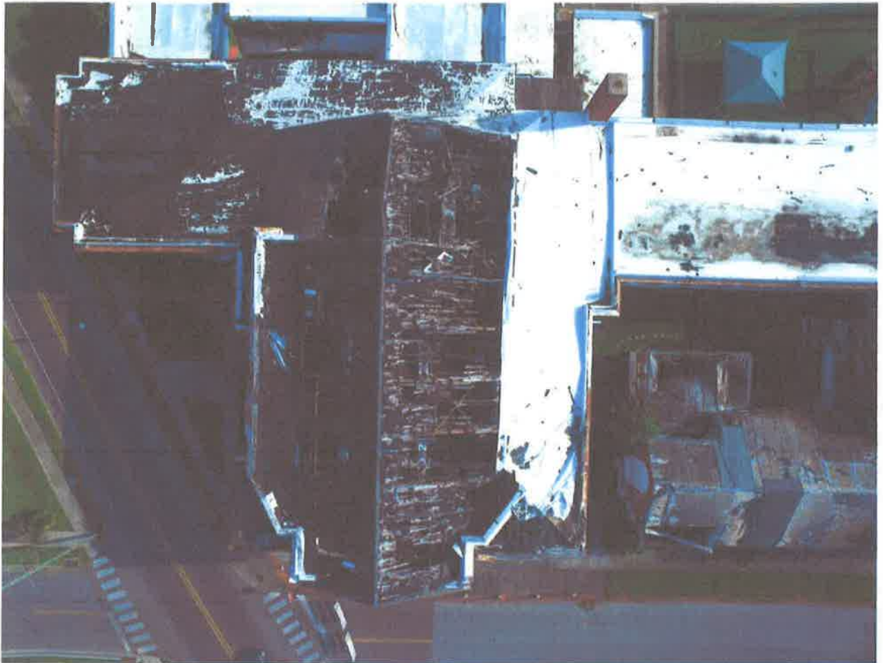
Figure 1 Aerial View of Overall Roof Condition
