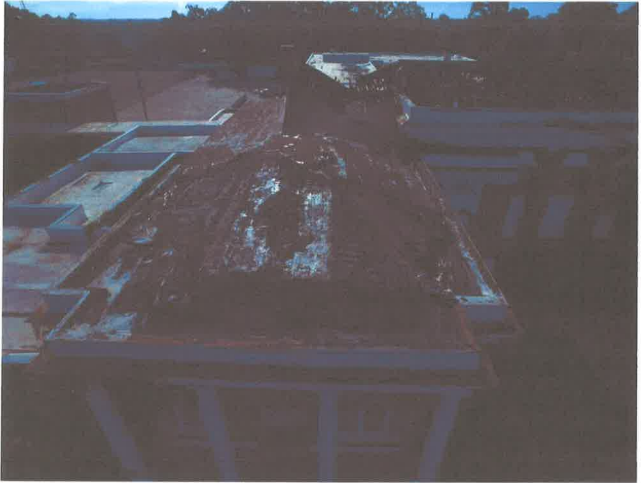
Figure 3 Roof Condition Northwest Corner Facing Main Street
